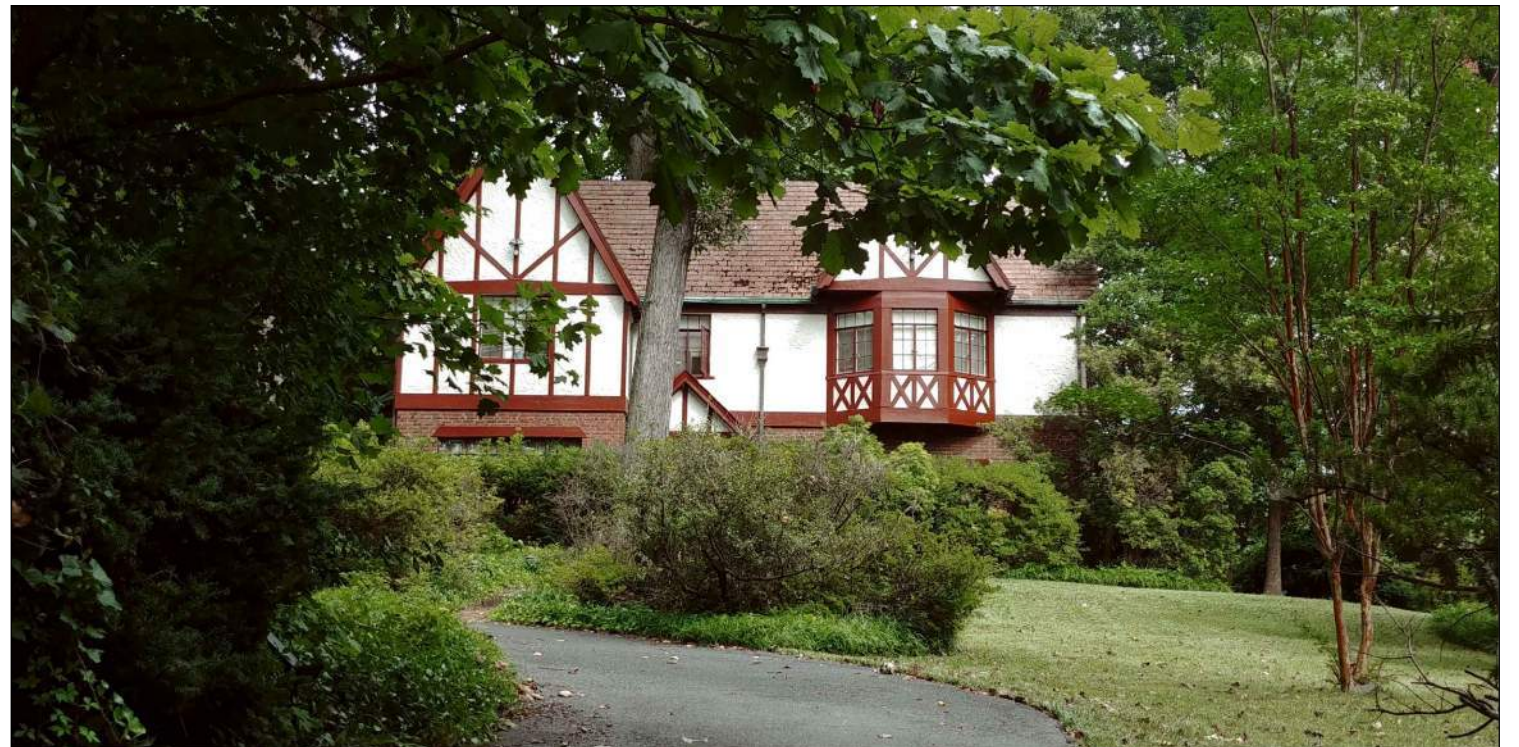
BRICK/STUCCO TUDOR REVIVAL HOUSE AT 7805 OVERHILL ROAD, PROVIDED AS A PRECEDENT FOR USE OF STUCCO AND HALF-TIMBERING OVER A BRICK BASE ON ADDITION
