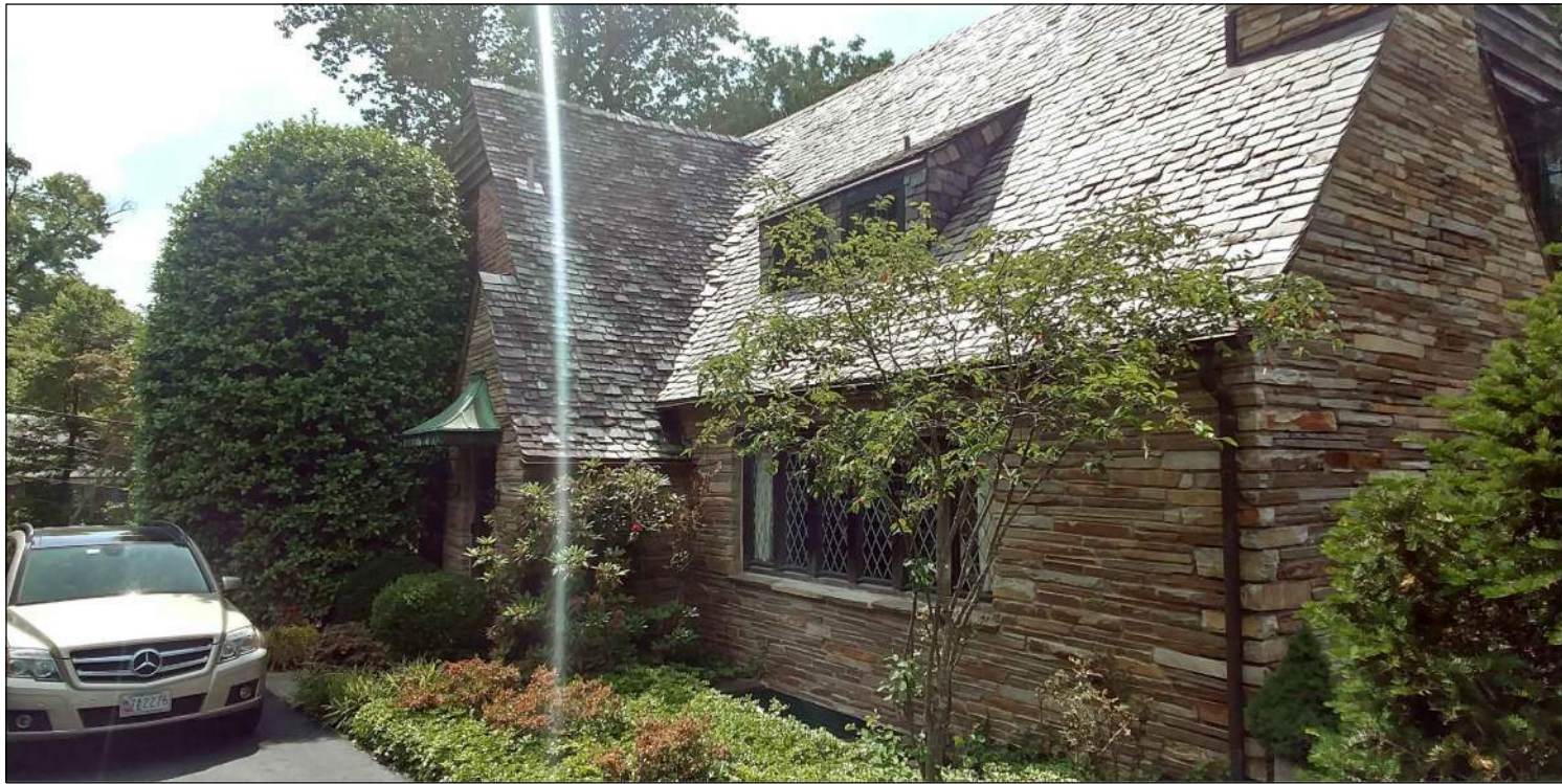
ADDITIONAL FRONT ELEVATION VIEW, NOTE DIAMOND MUNTIN WINDOWS AND COPPER ROOFING USED AS PRECEDENT FOR DETAILS ON ADDITION
