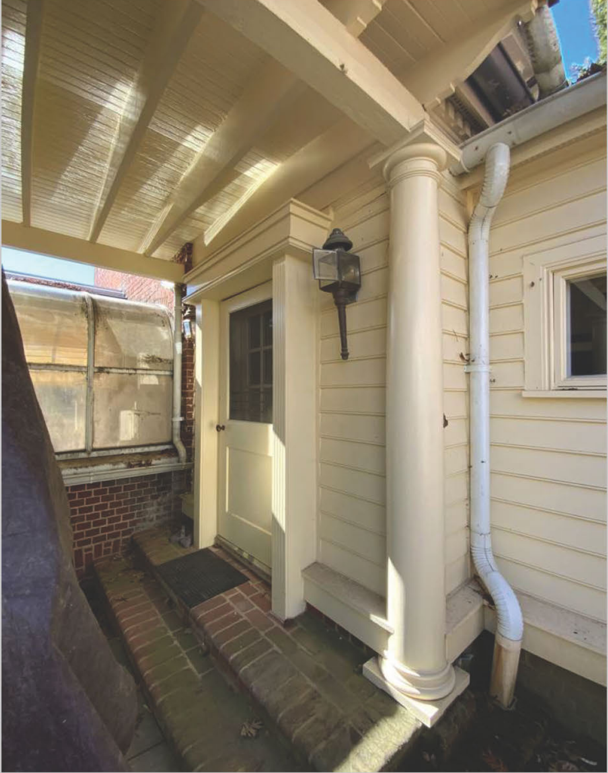
EXISTING ENTRY TO FIRST FLOOR KITCHEN ADDITION (BUILT C. 1985)
