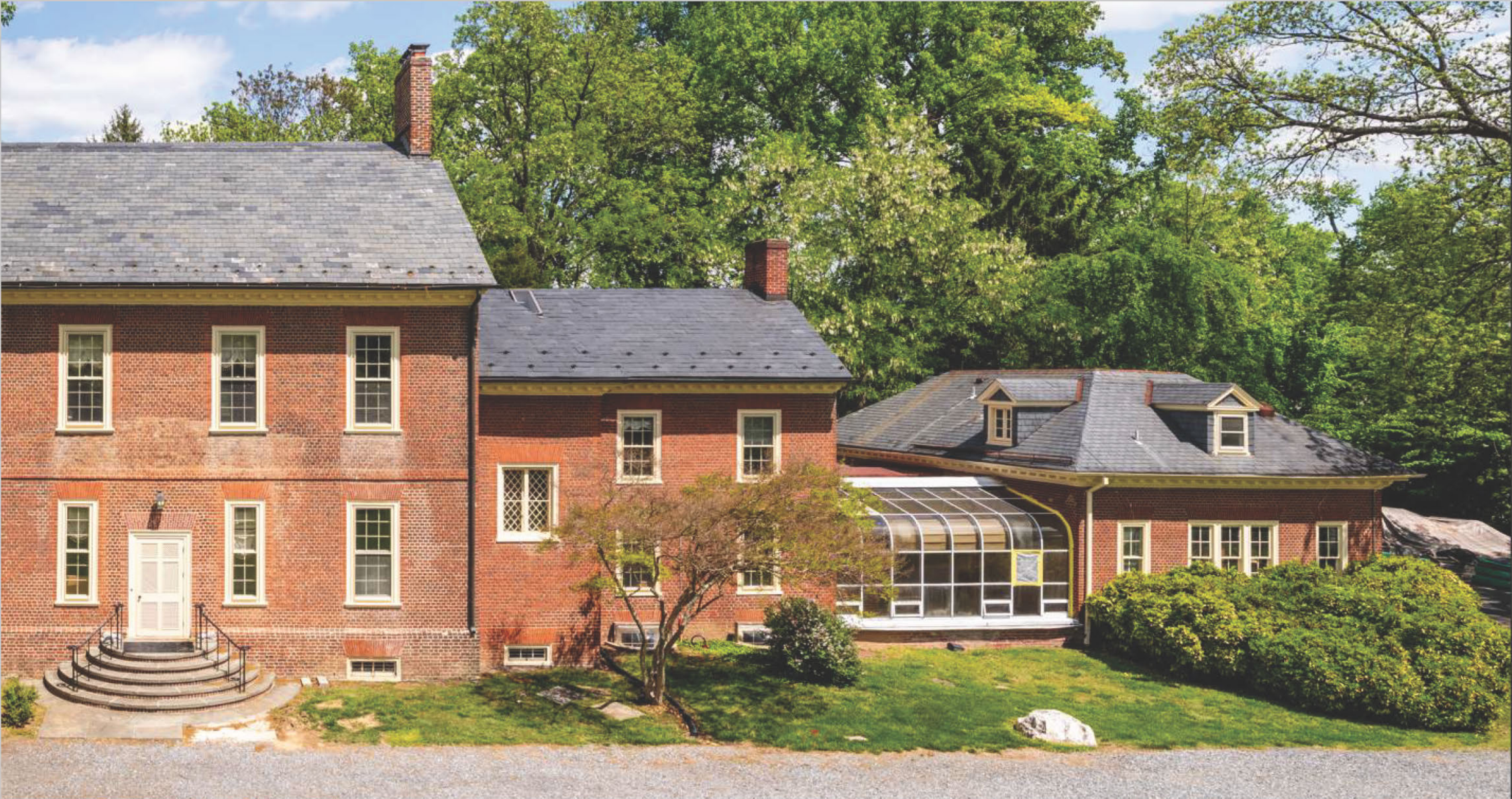
BIRDSEYE VIEW OF SOUTH FACADE WITH EXISTING GREENHOUSE AND GARAGE LOCATED EAST OF THE MANOR HOUSE
