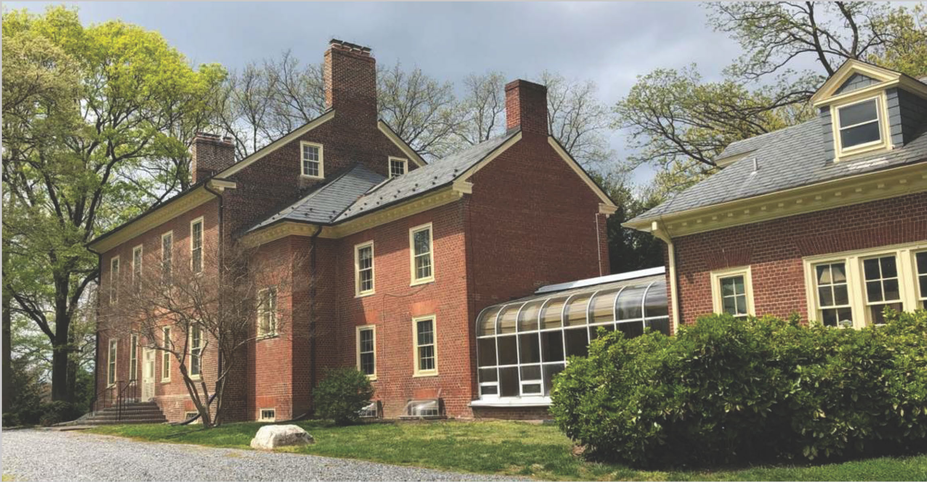
SOUTHEAST VIEW OF SOUTH FACADE WITH EXISTING GREENHOUSE AND GARAGE LOCATED AT THE RIGHT, EAST OF THE MANOR HOUSE
