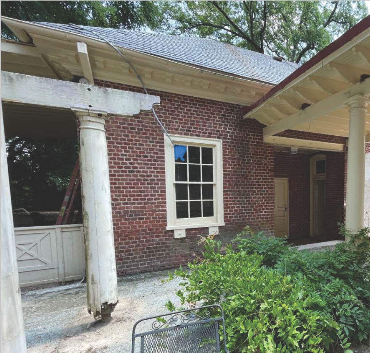
NORTHWEST VIEW OF GARAGE, WINDOW TO BE MODIFIED TO PROVIDE ENTRY TO GARAGE
