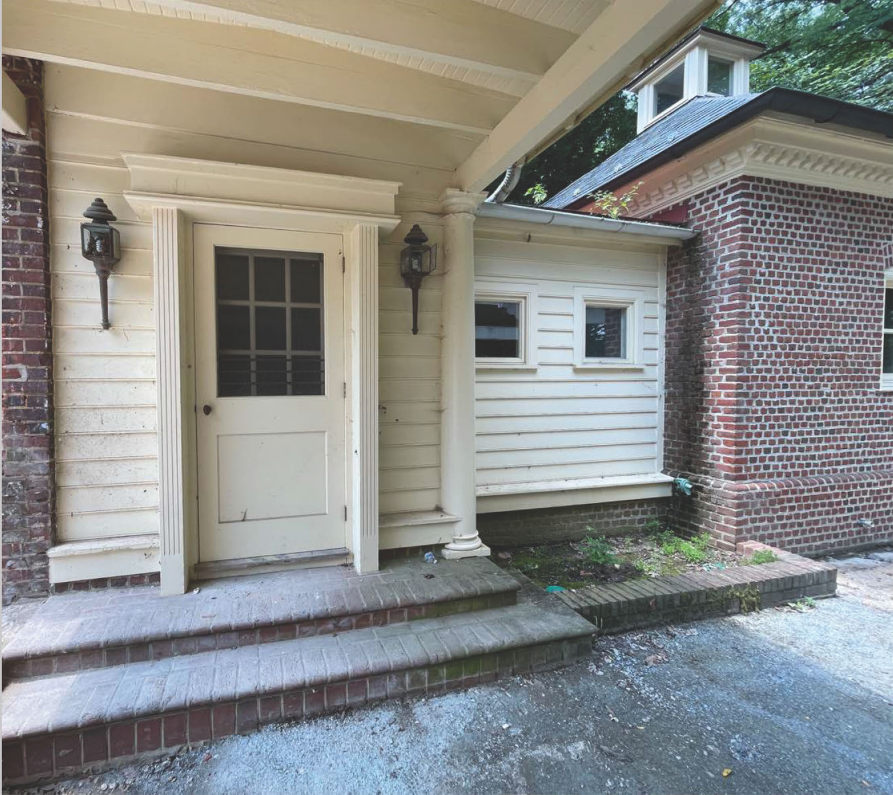
EAST VIEW OF EXISTING FIRST FLOOR KITCHEN ADDITION (BUILT C. 1985)
