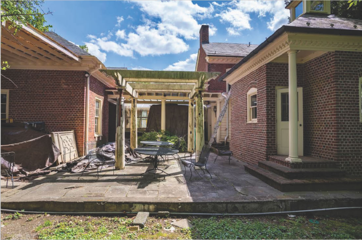
NORTH VIEW OF EXISTING EAST PATIO
