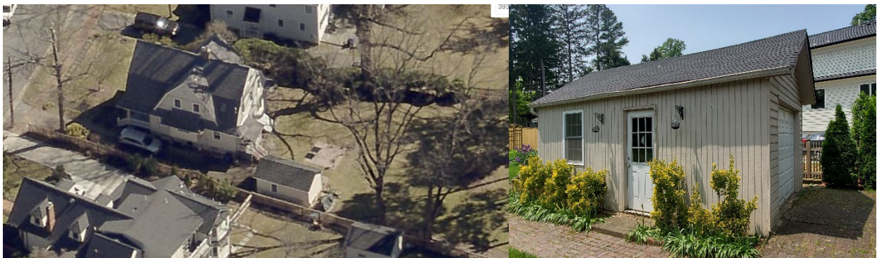
Figure 3: Aerial view from the west of property (left) and view of the north and east elevation of the detached garage (right).
