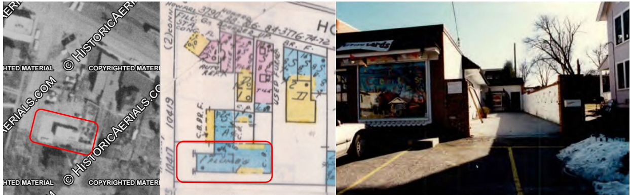
Figure 3: Historic views of the subject property at 10417 Armory Avenue. The aerial (left) shows the building prior to the construction of the additions to the north and east. The 1950-1963 Sanborn Fire Insurance Map (center) showing the subject property. A 1996 photograph (right) of the courtyard on the right shows the courtyard prior to the approval of the wrought-iron gates.
