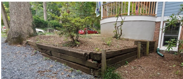
Figure 3: View of the existing retaining wall to be removed.
