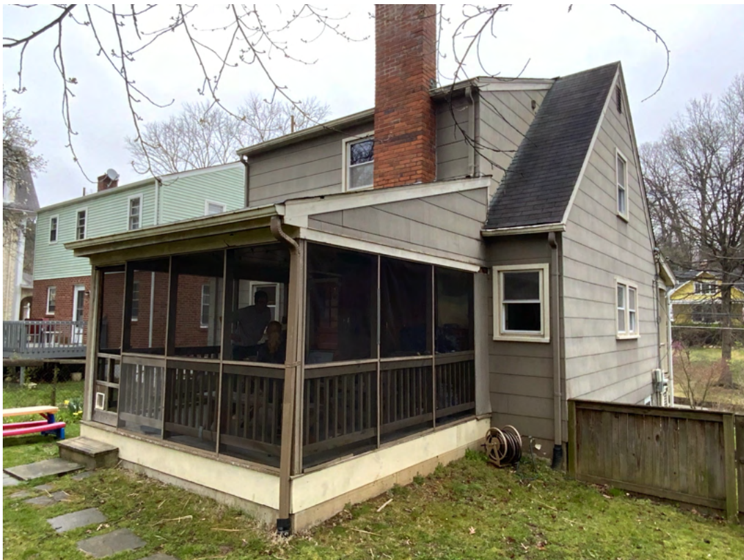
Detail: 7102 POPLAR SOUTH-EAST CORNER
