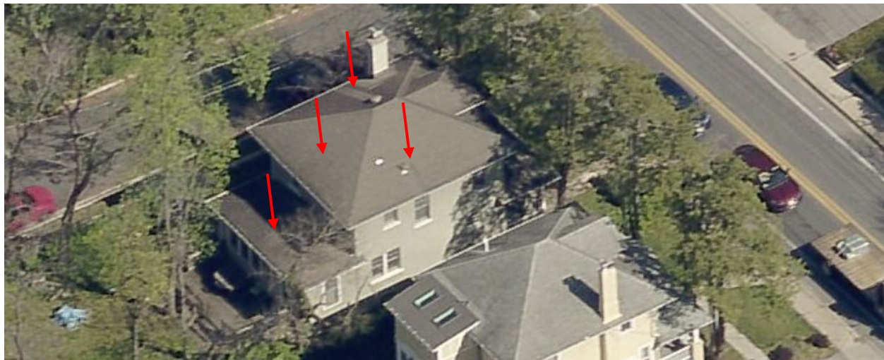
Figure 3: Aerial view, 2022. The red arrow points to the locations of the proposed arrays. Please note that a recently approved HAWP moved the roof vents after this aerial photograph.
