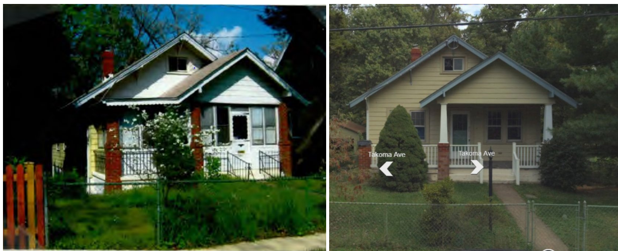
Figure 2: View of the subject property at 7305 Takoma Avenue, 2008 and 2014. Source: Montgomery Planning and Microsoft Bing Maps.
