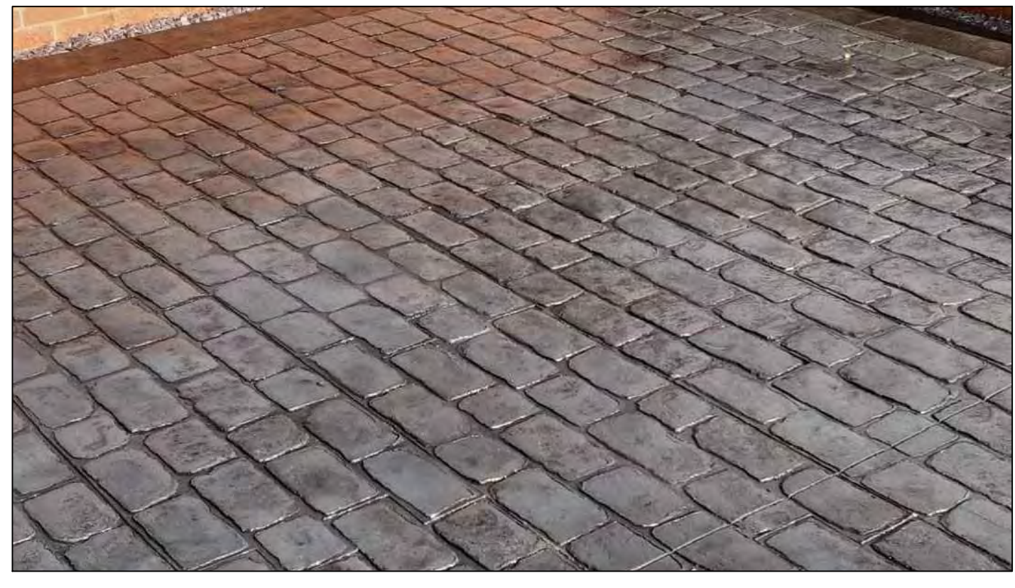
PRESSED CONCRETE INSTALLED EXAMPLE
