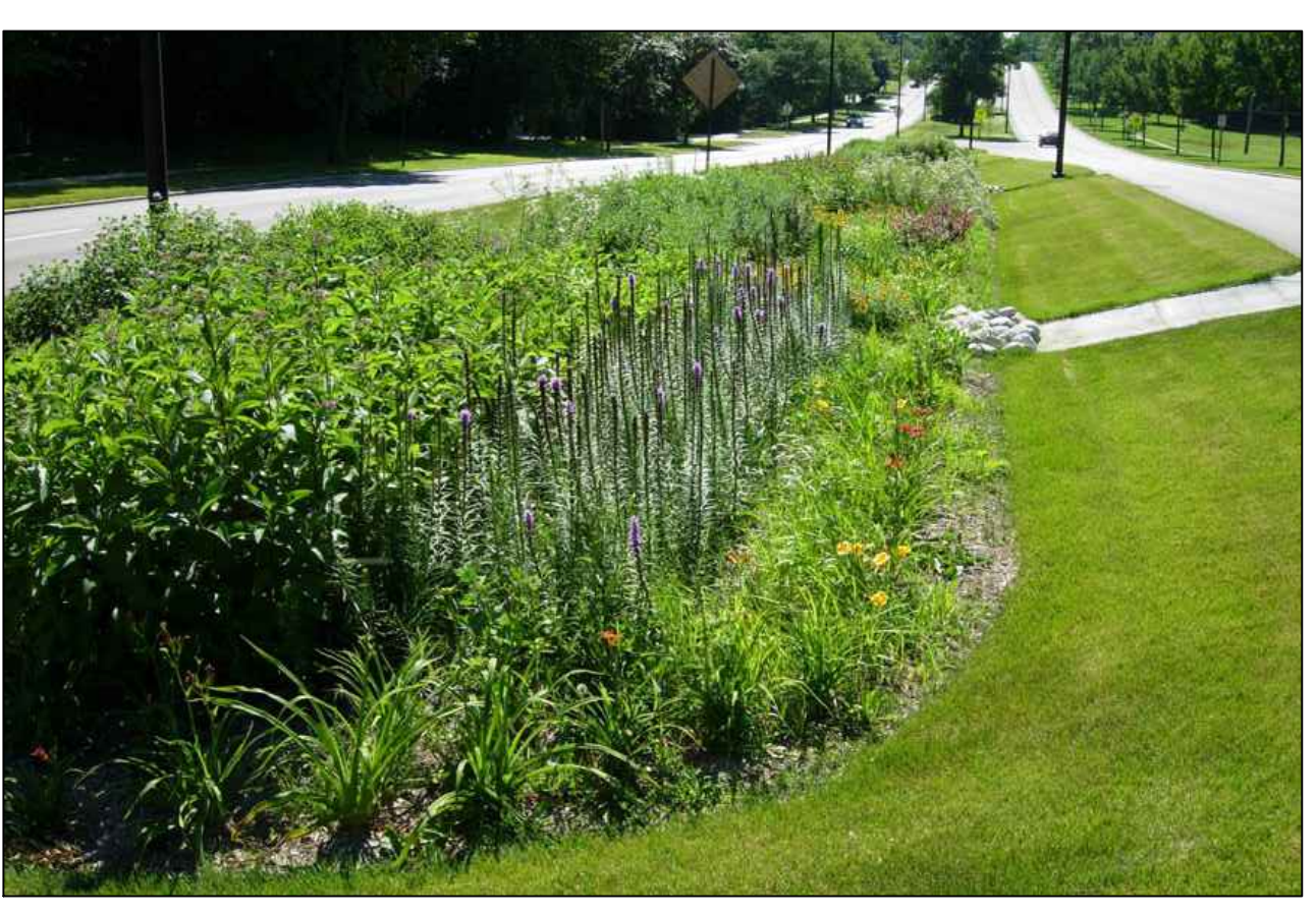
BIO-SWALE INSTALLED EXAMPLE
