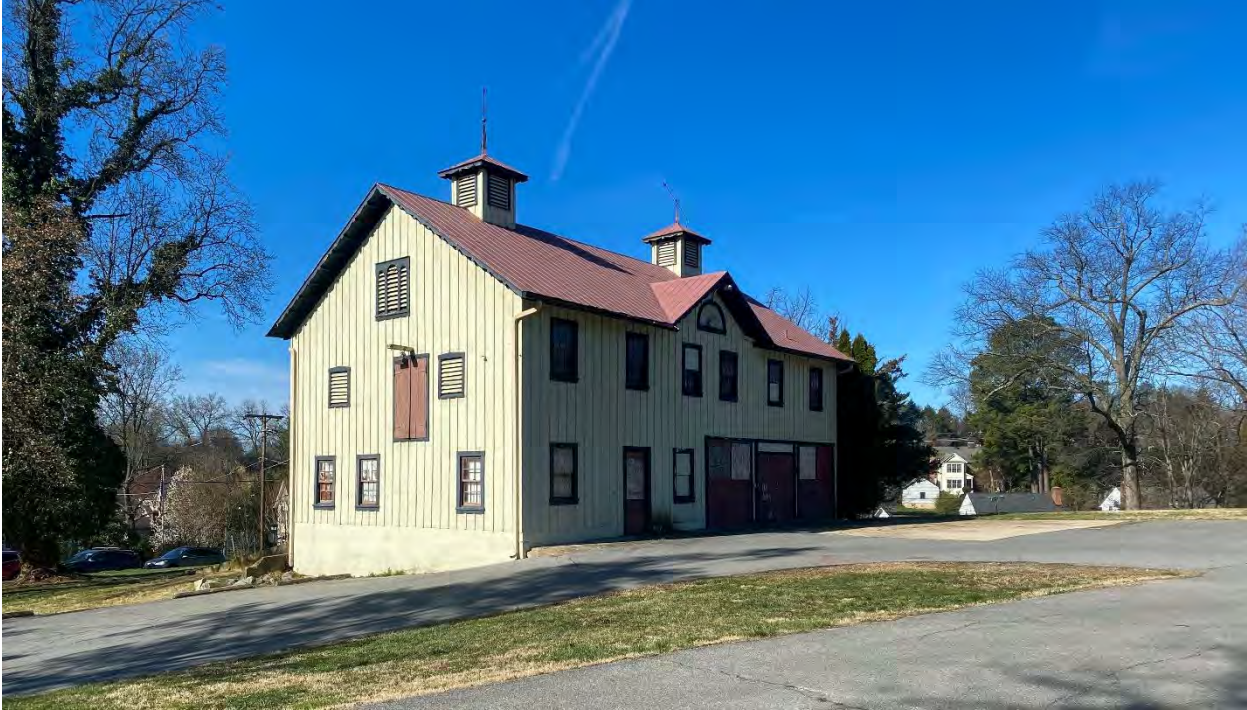
Figure 9: 2023 image of the carriage house.
