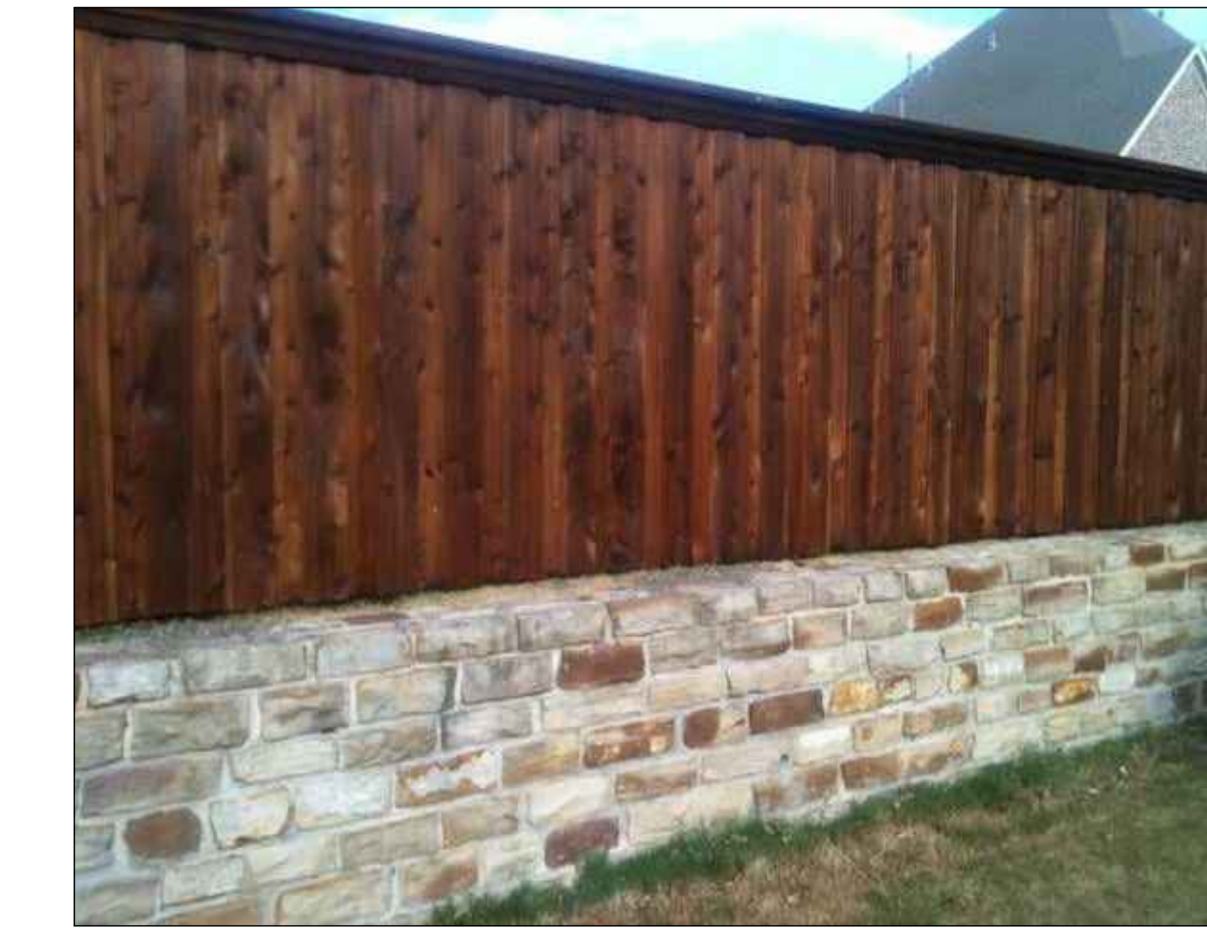
DUMPSTER WALL WITH FENCE INSTALLED EXAMPLE
