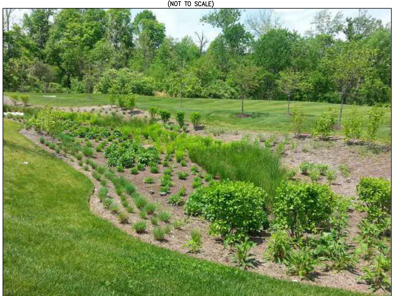
MICRO-BIORETENTION INSTALLED EXAMPLE
