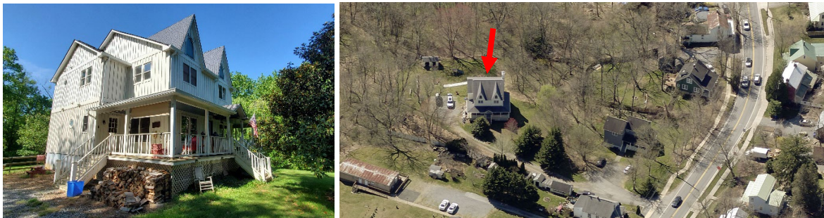
Figure 2: View of the north and east elevations, 2023 (left), and aerial view showing the subject house (red arrow) in relation to Frederick Road (right).
