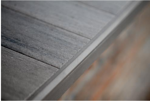
Figure 2: The chamfer nosing trim piece can cover the exposed ends of the tongue and groove flooring.
