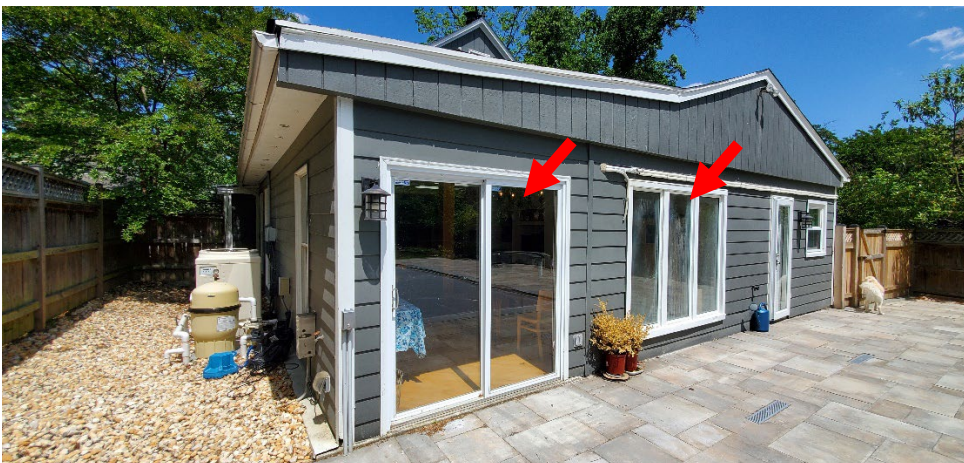
Figure 3: View of the rear elevation of the non-contributing house, 2023. The two red arrows point to the door and windows to be replaced by double-leaf, fiberglass doors. The cementitious fiberboard lap siding on the entire rear elevation would be replaced in-kind. Source: Montgomery Planning.
