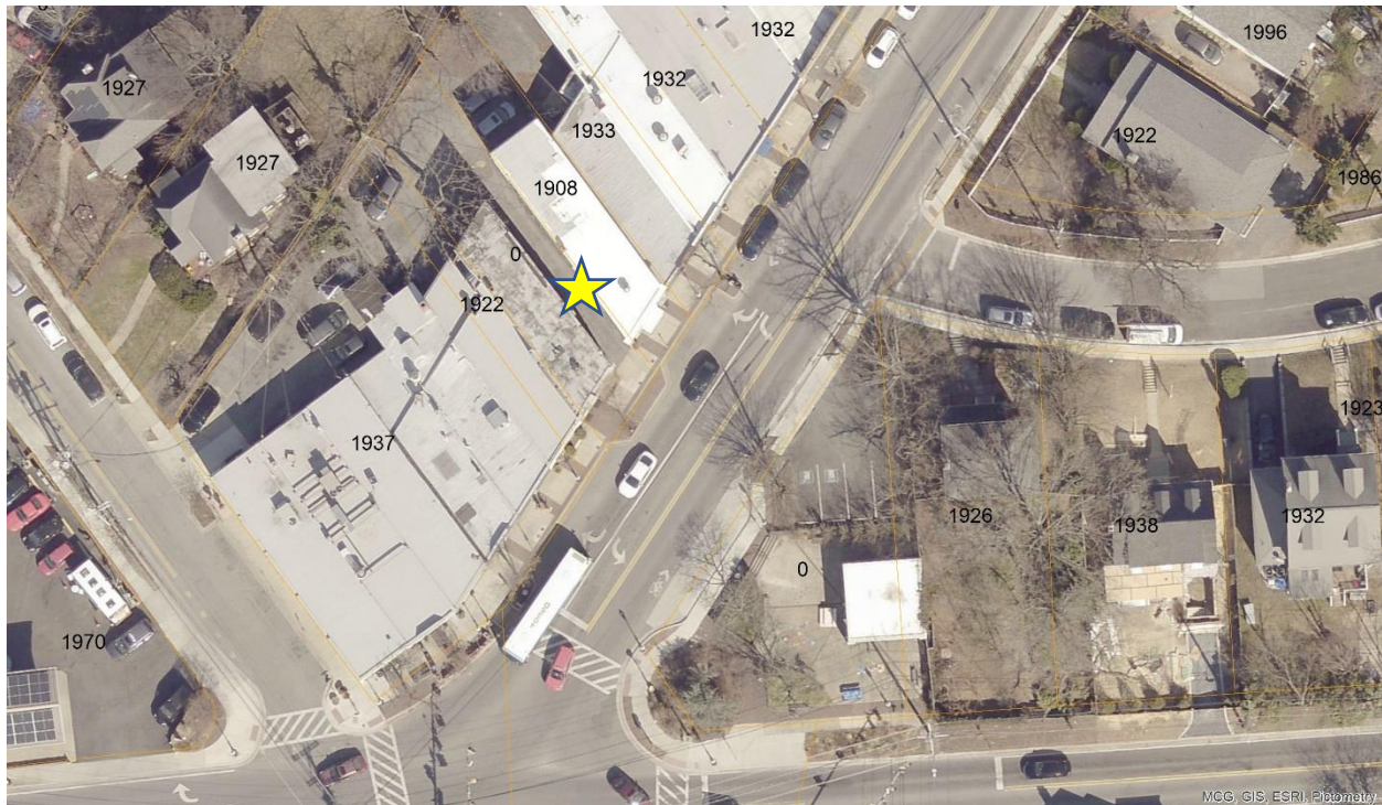
Figure 1: The subject property, identified by the yellow star, is located on the west side of Carroll Avenue and adjacent to a narrow alley.
