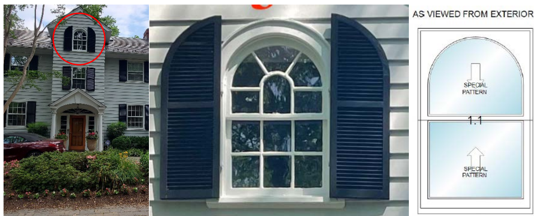
Figure 3: View of the façade of 45 West Lenox Street, 2023 (left), close-up view of Window #3 (middle), and applicant's proposed replacement specification labeled as “ultra rectangular out – half circle in double hung” (right). Source: Montgomery Planning and Applicant.
