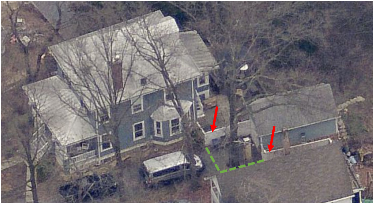
Figure 2: Detailed view of the existing privacy fence noted by the red arrows. The green dashed line is the proposed location for the new fence which encloses the garage in the rear yard.
