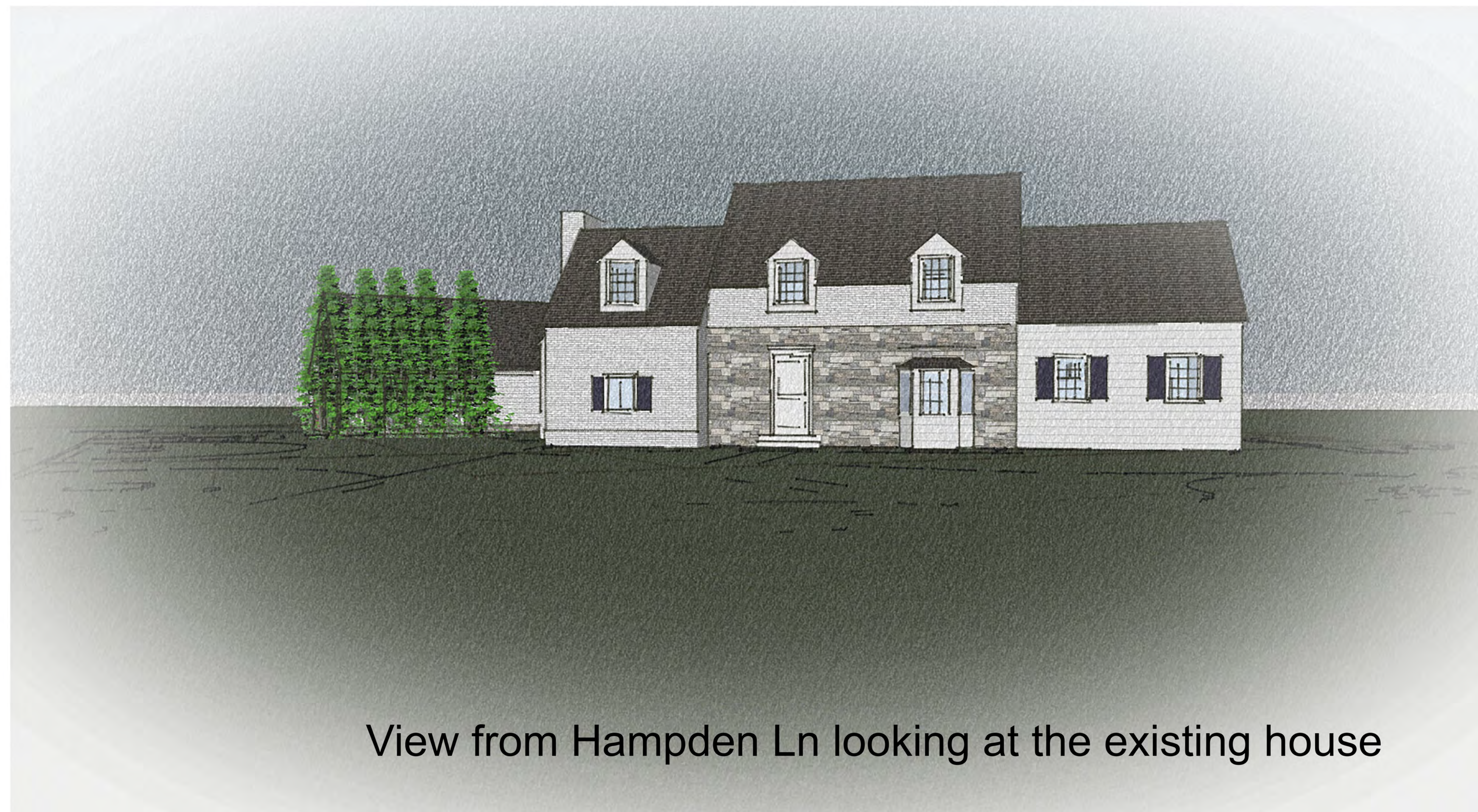
View from intersection of Hampden Ln and York Ln
