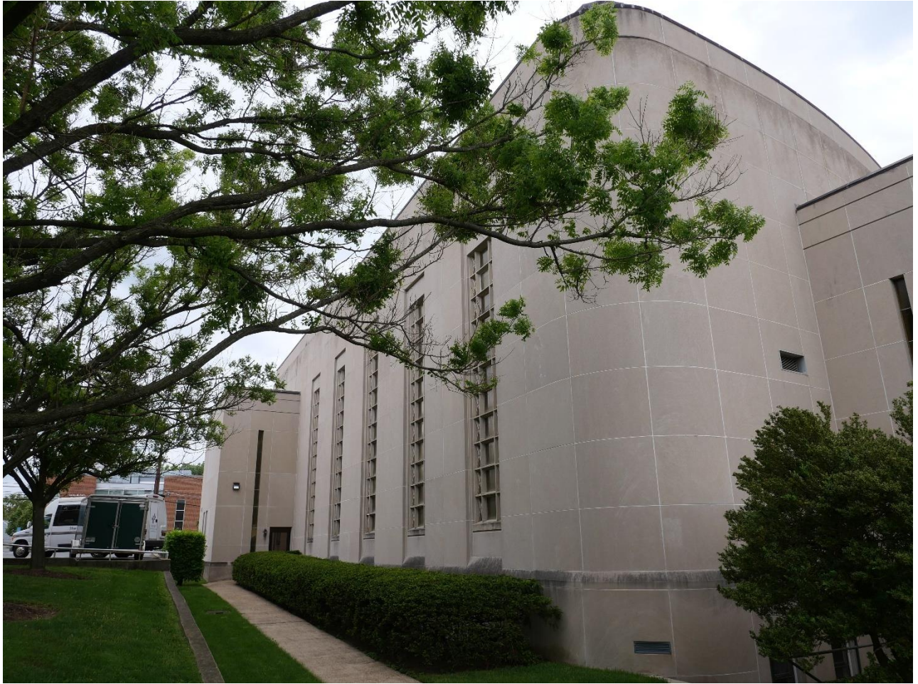
Figure 7: West elevation, viewed from southwest corner. Source: Montgomery Planning
