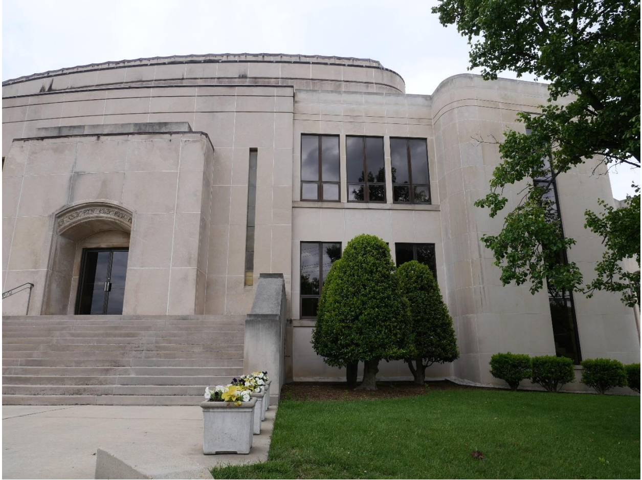
Figure 10: A three-bay hyphen connects the 1985 addition to the original façade (south elevation). Source: Montgomery Planning.
