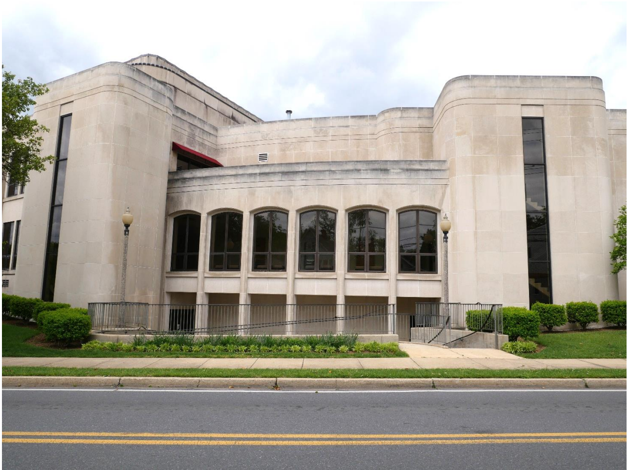
Figure 9: 1985 addition, stairwells and central pavilion, looking north. Source: Montgomery Planning.
