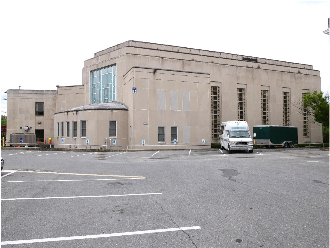
Figure 6: West and north (rear) elevations, looking south. Source: Montgomery Planning.
