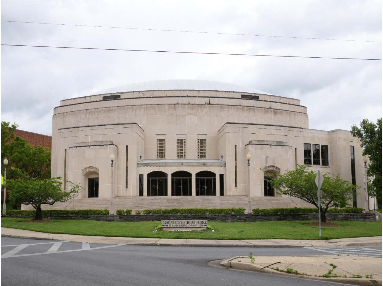
Figure 1: South elevation, looking northeast. Source: Montgomery Planning.
