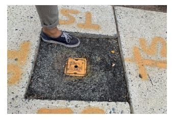
A poorly filled utility cut in the sidewalk. Shoe for scale.
