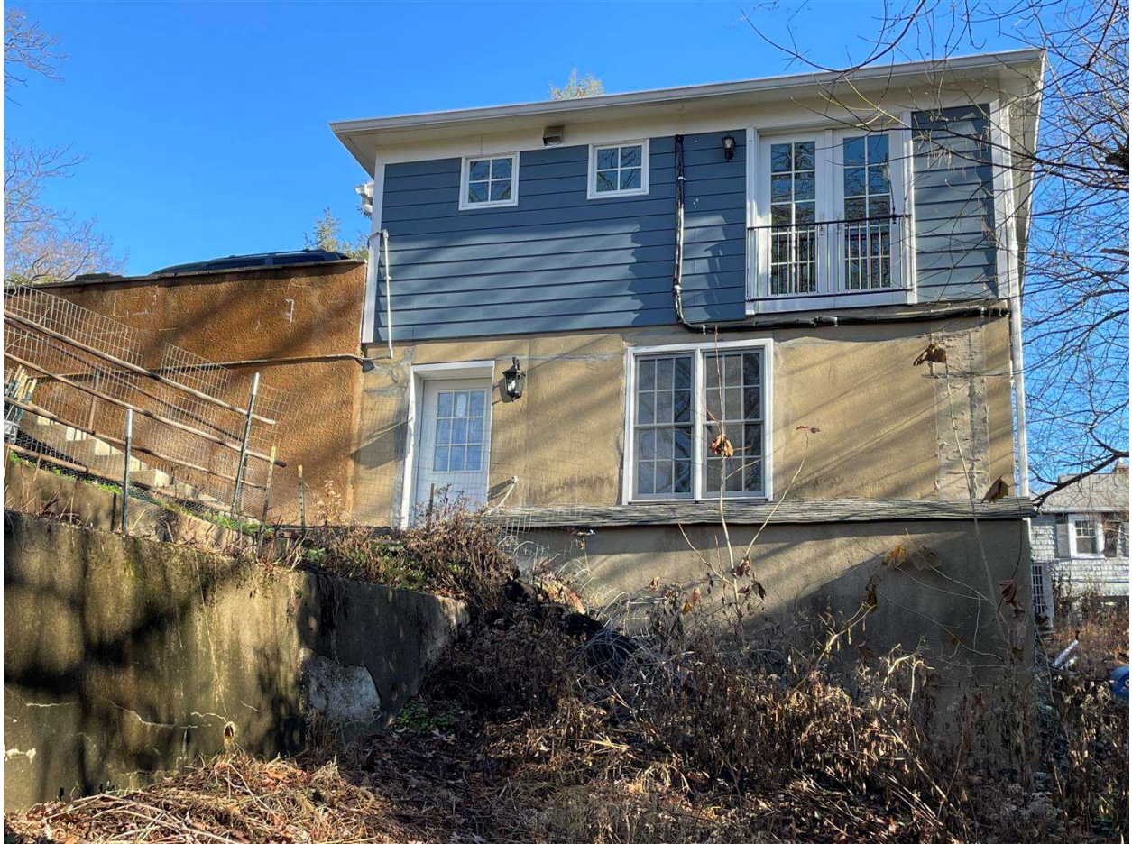
Figure 10: West elevation of the former garage from terraced yard, view to east, Nancy LiPira, December 9, 2022.
