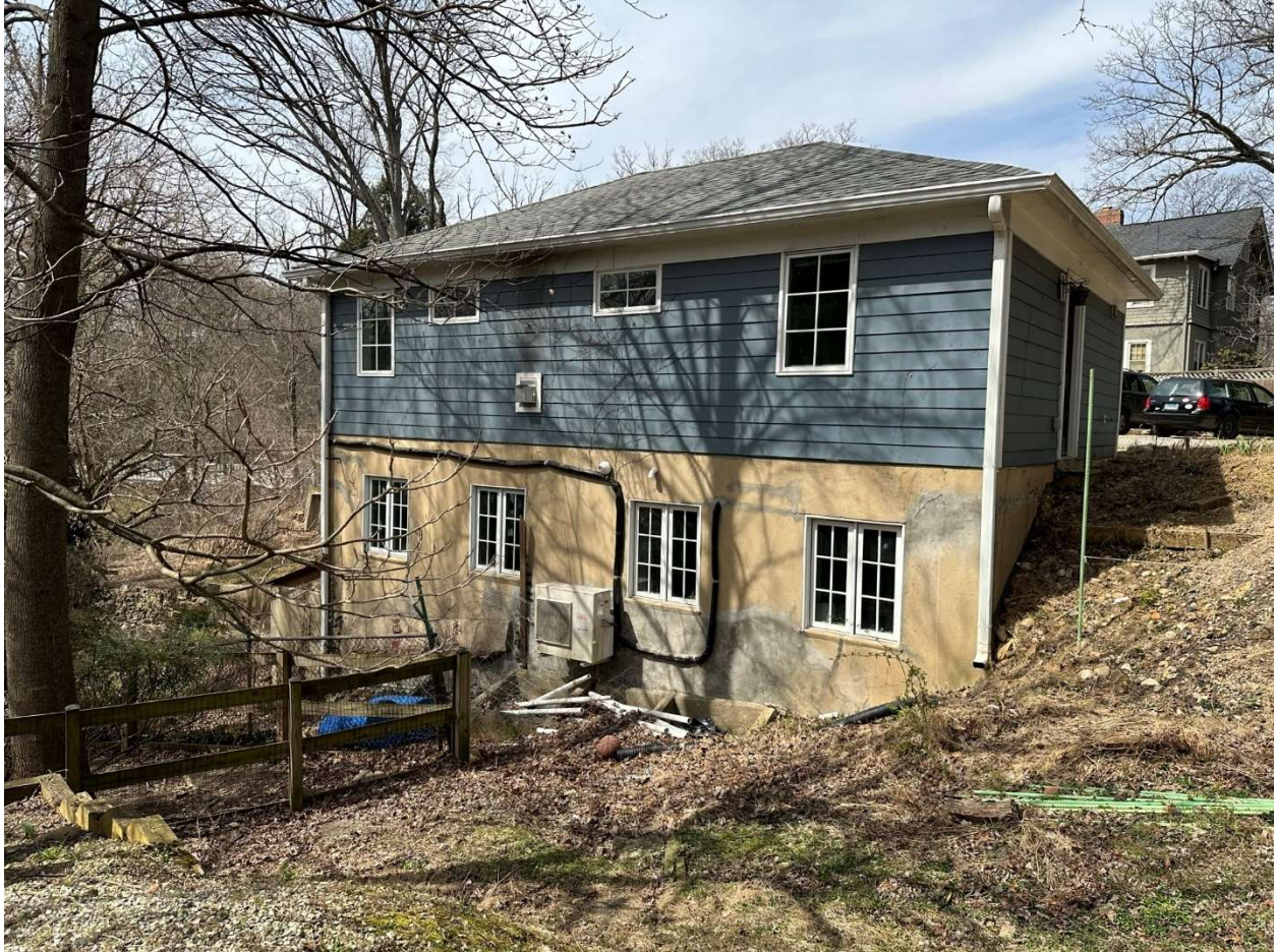
Figure 11: Southeast corner of the former garage. Montgomery Planning, March 22, 2023.
