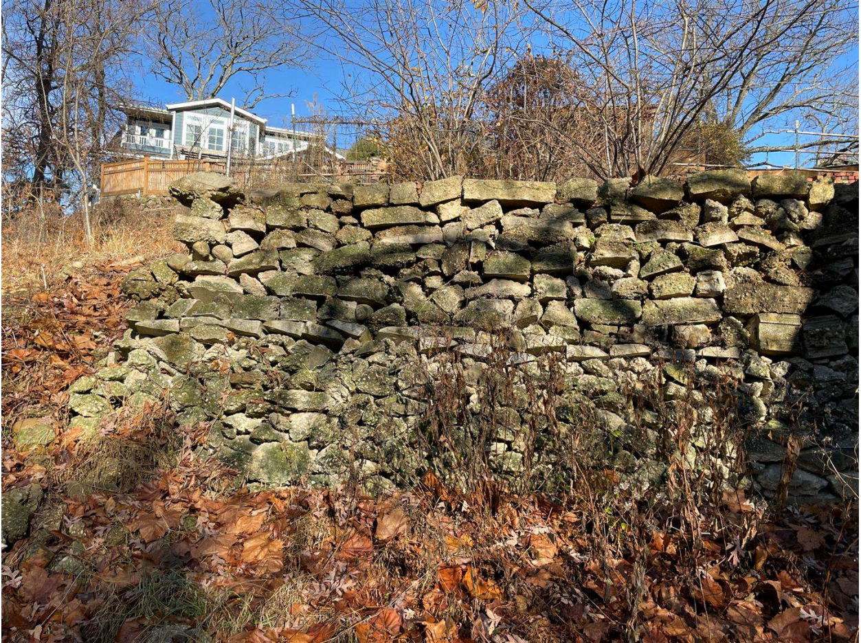
Figure 13: Example of a dry-laid masonry retaining wall in terraced rear yard, Nancy LiPira, December 9, 2022.
