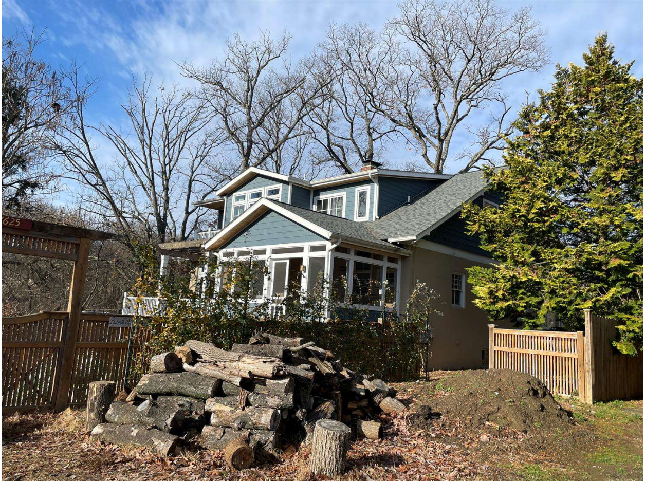
Figure 4: South (rear) elevation of the Kress House showing recent alterations, view to northwest, Nancy LiPira, December 9, 2022.
