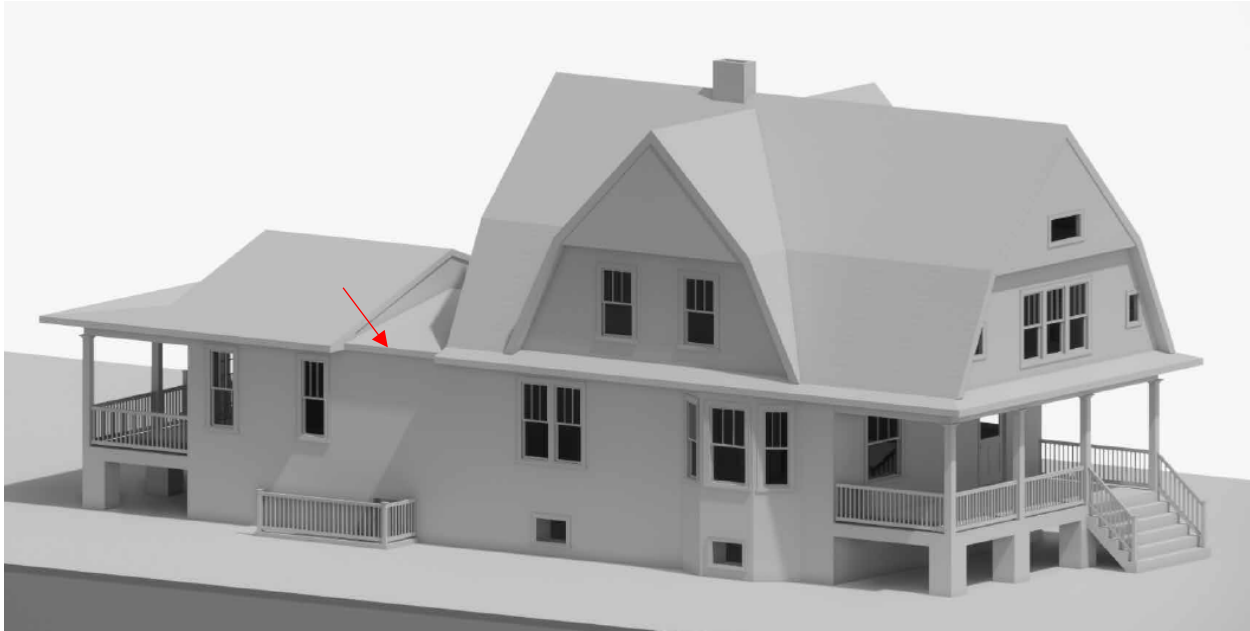
Figure 5: View of the east (side elevation). Note the recessed eave line of the addition (red arrow).
