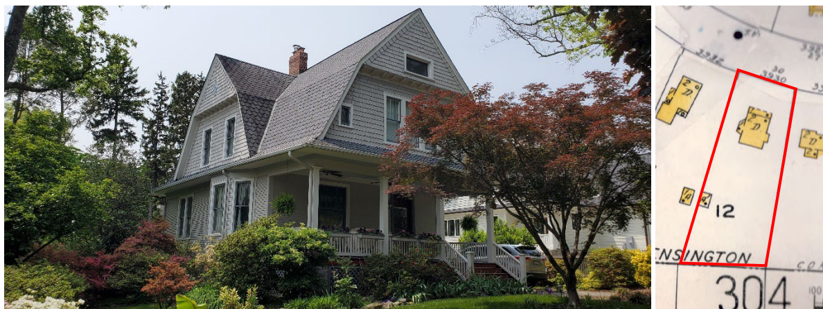
Figure 2: View of the façade (north) and east elevation of the subject house (left) and the 1950-1963 Sanborn Fire Insurance Map (property outlined in red).
