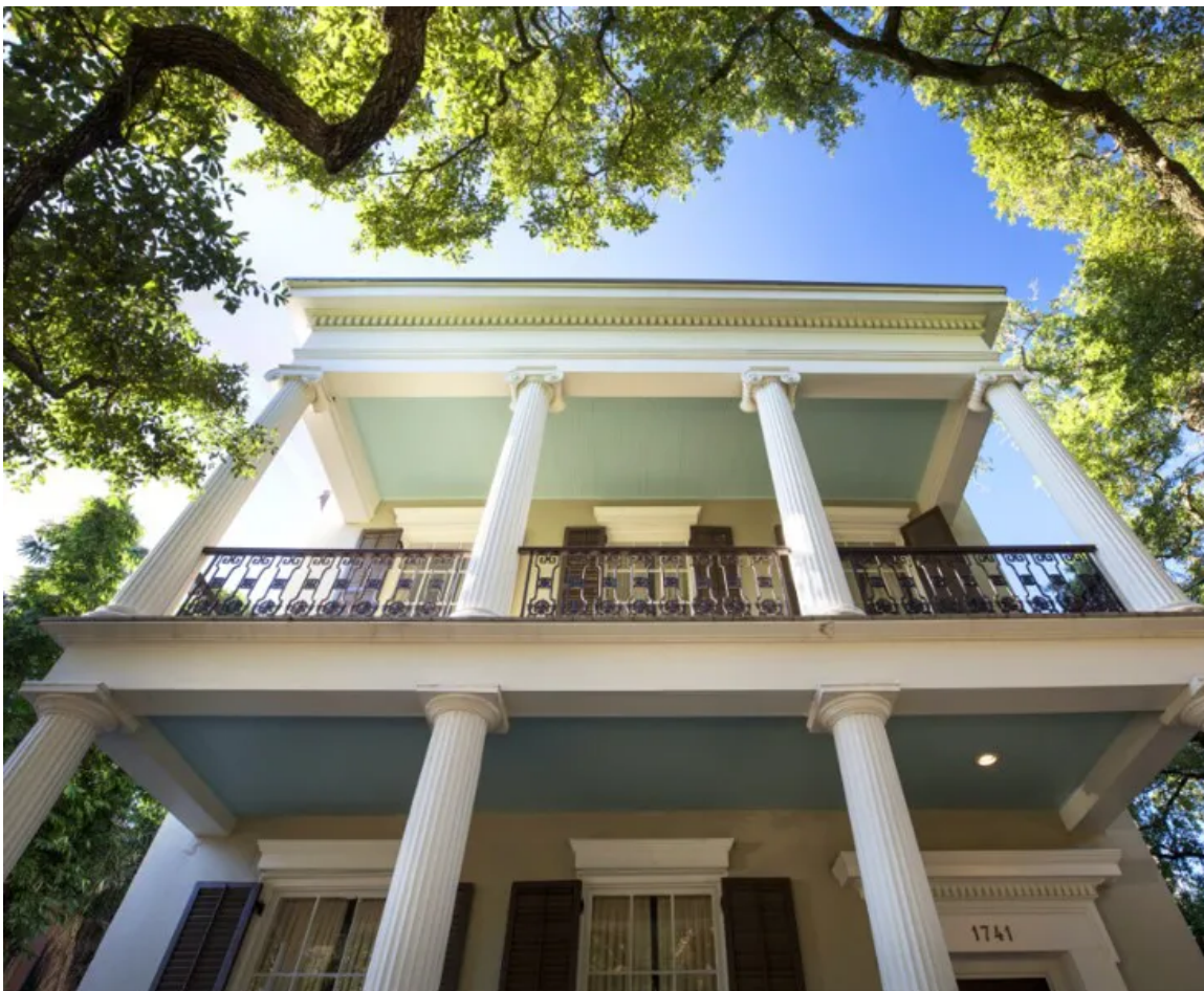
Photo courtesy of Aeratis
