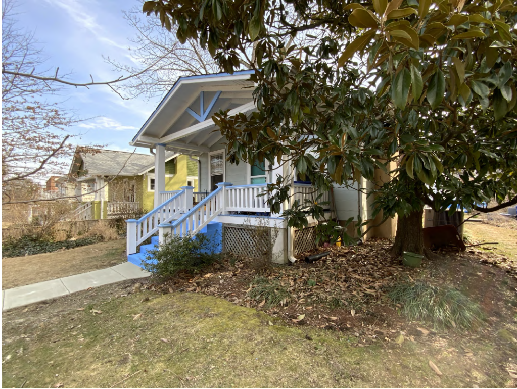
Detail: 109 ELM PORCH NORTHWEST CORNER
