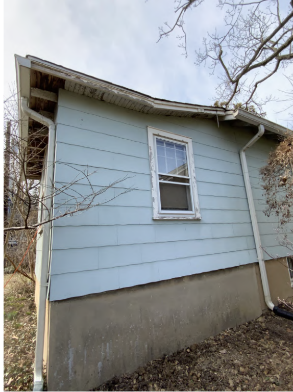
Detail: 109 ELM REAR SOUTHEAST CORNER
