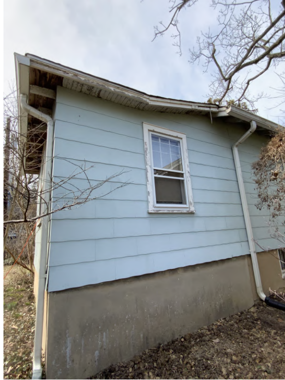
Detail: 109 ELM REAR SOUTHEAST CORNER
