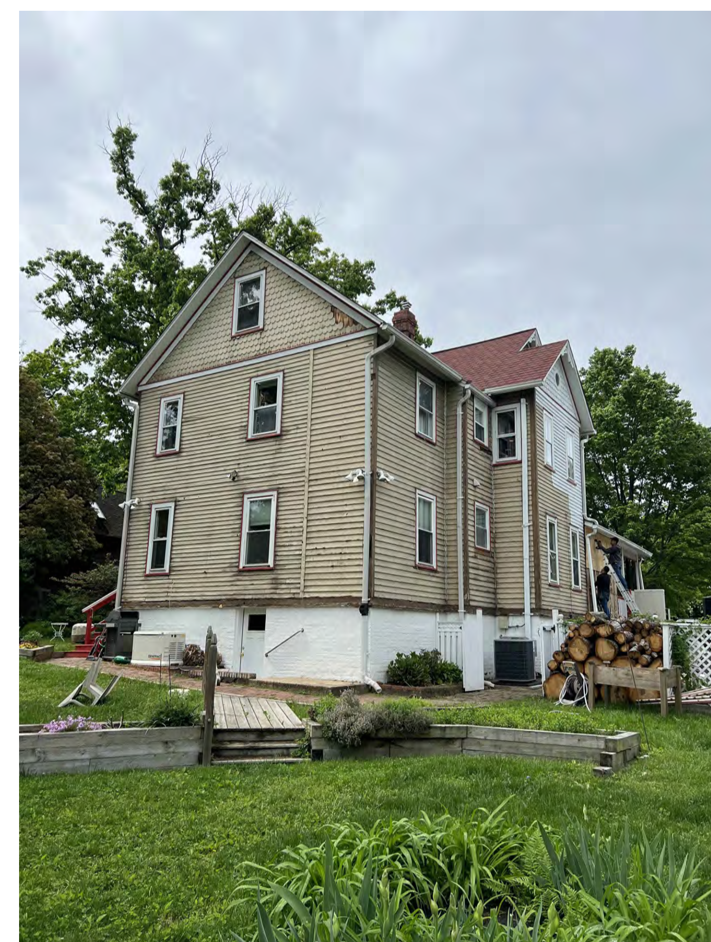
Existing conditions looking at South(Back) and East(Side) Facades
