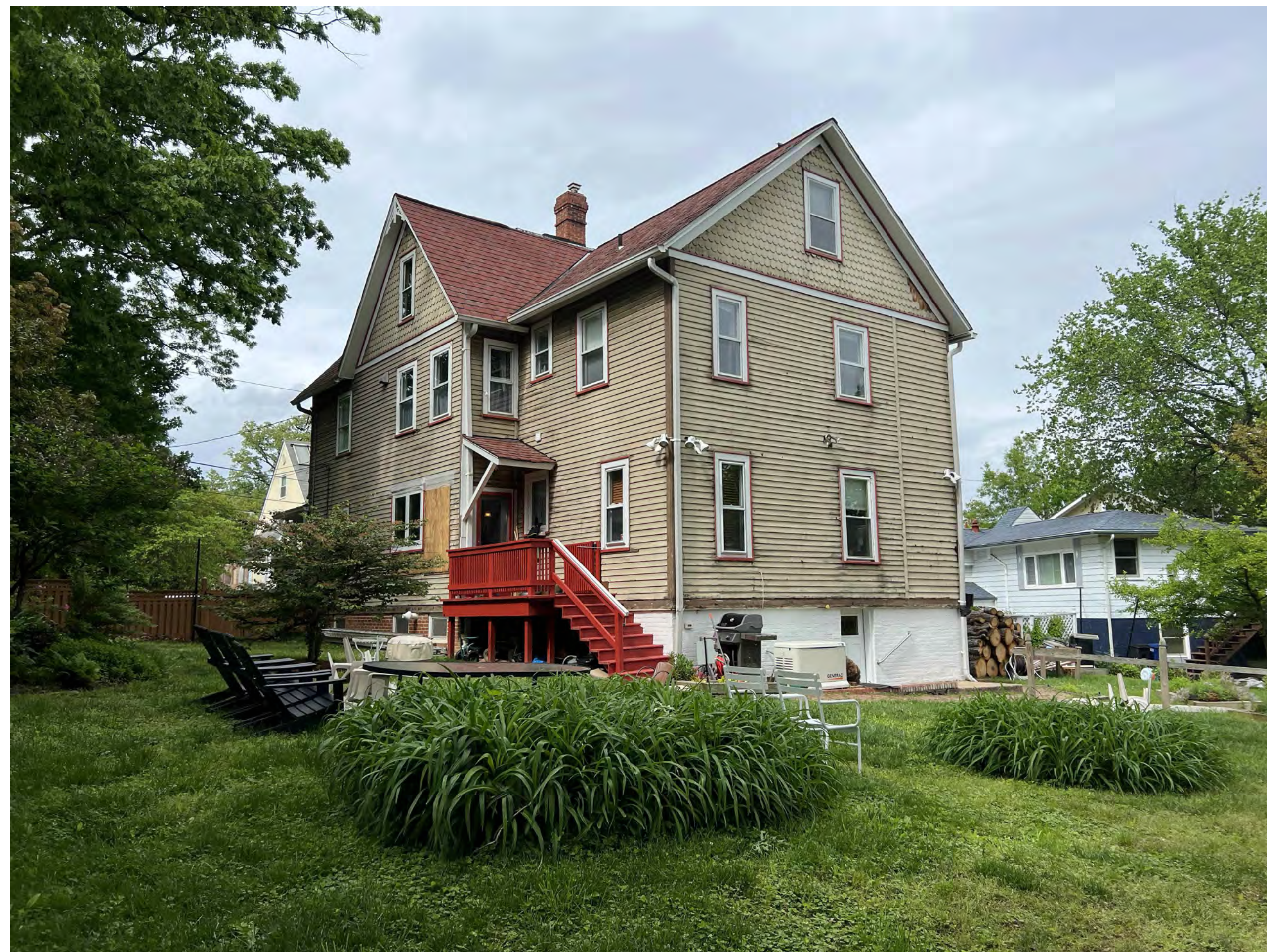
Existing conditions looking at South(Back) and West(Side) Facades
