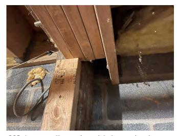
11B. Incorrectly centered 6x6 wood column and girder at 1890's block basement south wall.
