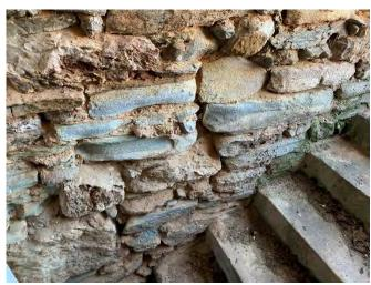
**7C**. Deteriorated mortar joints at 1797 block south basement entry wall.
