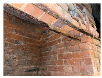
9B. Corroded and sagging wrought iron bars at basement firebox.
