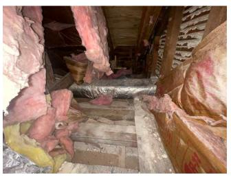
16. Missing floor and wall insulation in Room 307.
