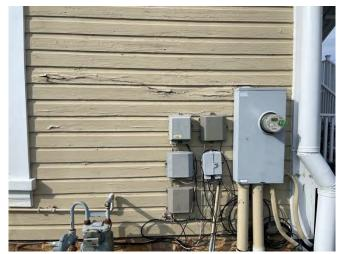
3A. Deteriorated clapboards at east facade.
