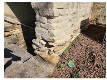
**7A**. Missing stone and deteriorated mortar joints at 1797 block south basement entry wall.
