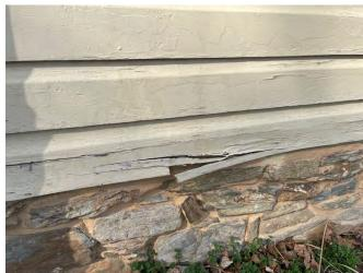
3B. Deteriorated clapboards at bottom of east facade.
