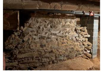
12. Partially collapsed stone wall at 1890's block basement west wall.
