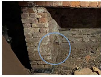
8. Deteriorated brick in 1797 block basement firebox.
