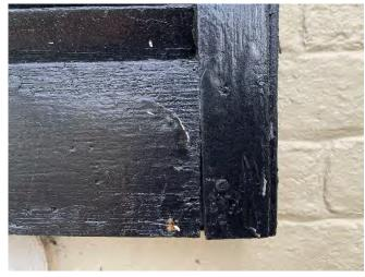
**6C**. Mortise-and-tenon joint with wood pegs of existing shutter.
