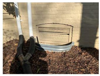
**5**. Broken wood louver at north (front) basement opening.
