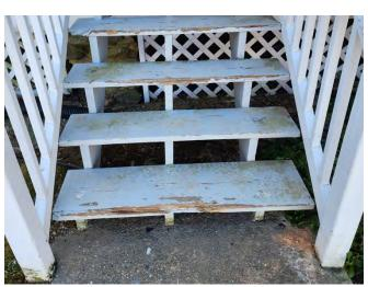
1B. Worn and cracked stair treads at north porch.
