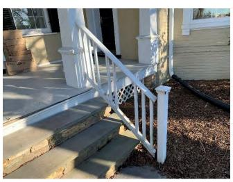
4. Deteriorated east side railing at 1797 block south (Front) porch
