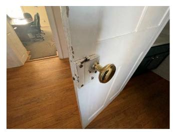
**22A**. Surface mounted cast-iron box lock at Room 105 door.
