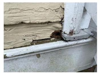
**3C**. Deteriorated clapboard at 1797 block north (rear) facade.
