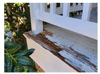
1A. Deteriorated floorboards and edge trim at porch corner.
