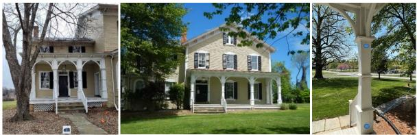
Figure 3: The subject porch posts, 2023 (left and center), and proposed location (blue circles) of vents on each column.
