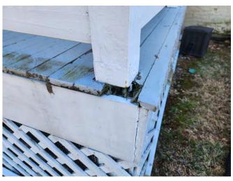
2. Deteriorating floorboards below north deck railing post.
