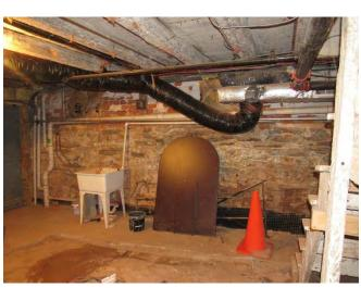
13. 1797 block log ceiling joists with no thermal insulation between joist.
