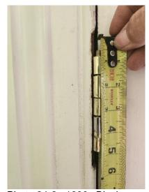
Photo 24-2: 1890s Block, Front Door Hinge
