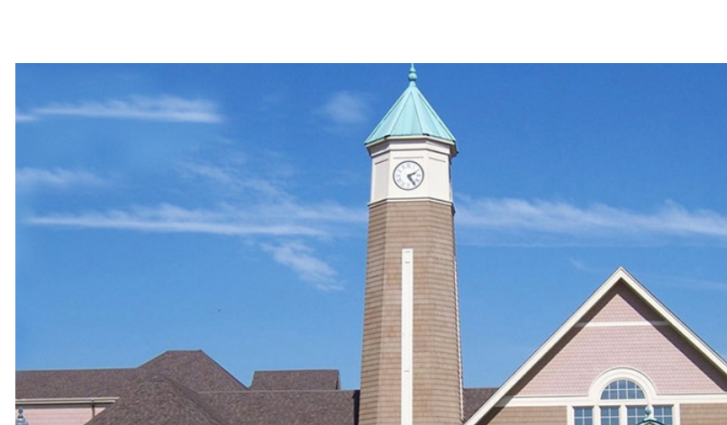
Project: The Glen Senior Living - Classic Residence by Hyatt Location: Chicago, IL Architect: Solomon Cordwell Buenz Co. - Chicago, IL Builder: JC Inc - Wheaton, IL Product: 7-1/8" Even Keyway Color: Rose Quartz & Taupe
