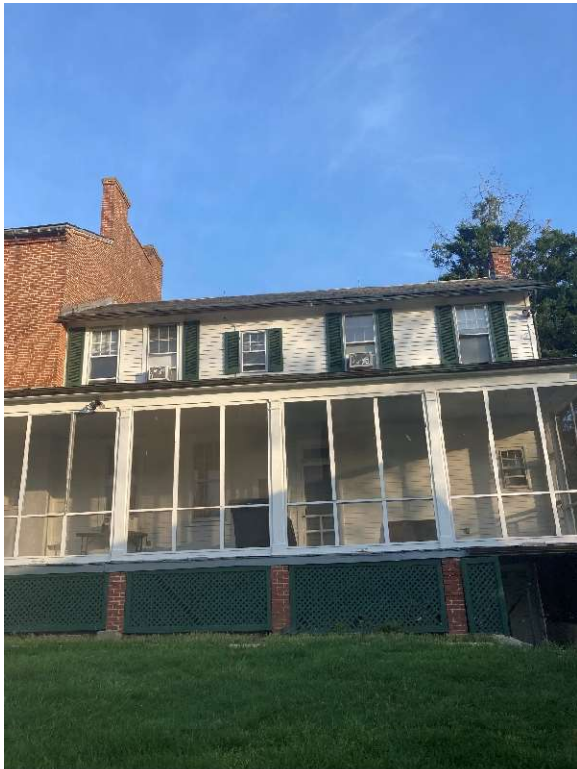
South (rear) elevation: 1913 addition
