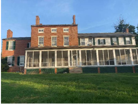
South (rear) elevation: main mass (center), 1913 addition (right) and 1954 addition (left)
