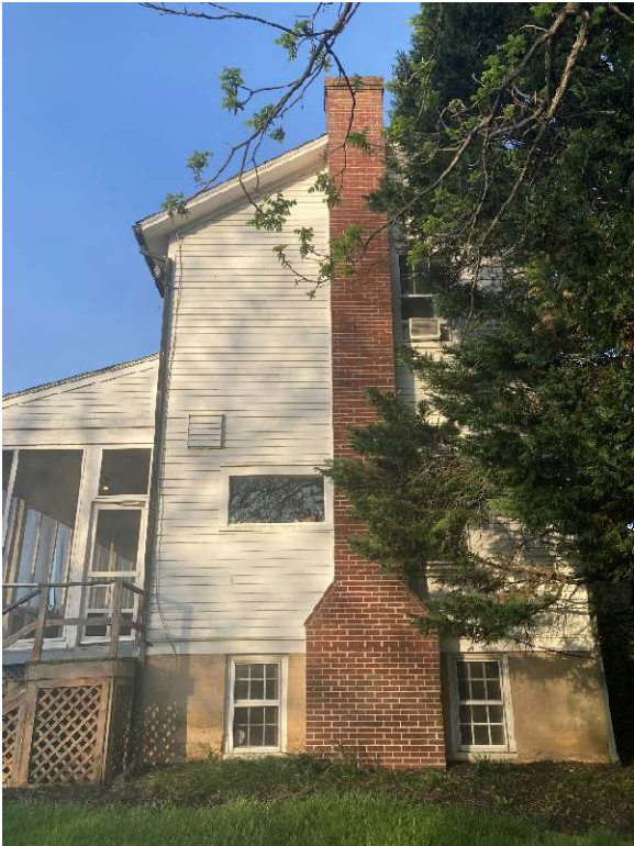
East elevation: 1913 addition
