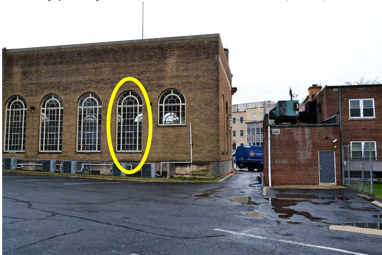
Figure 3: Rear of the subject property. The lower half of the window outlined in yellow will be removed to create access from the addition.
