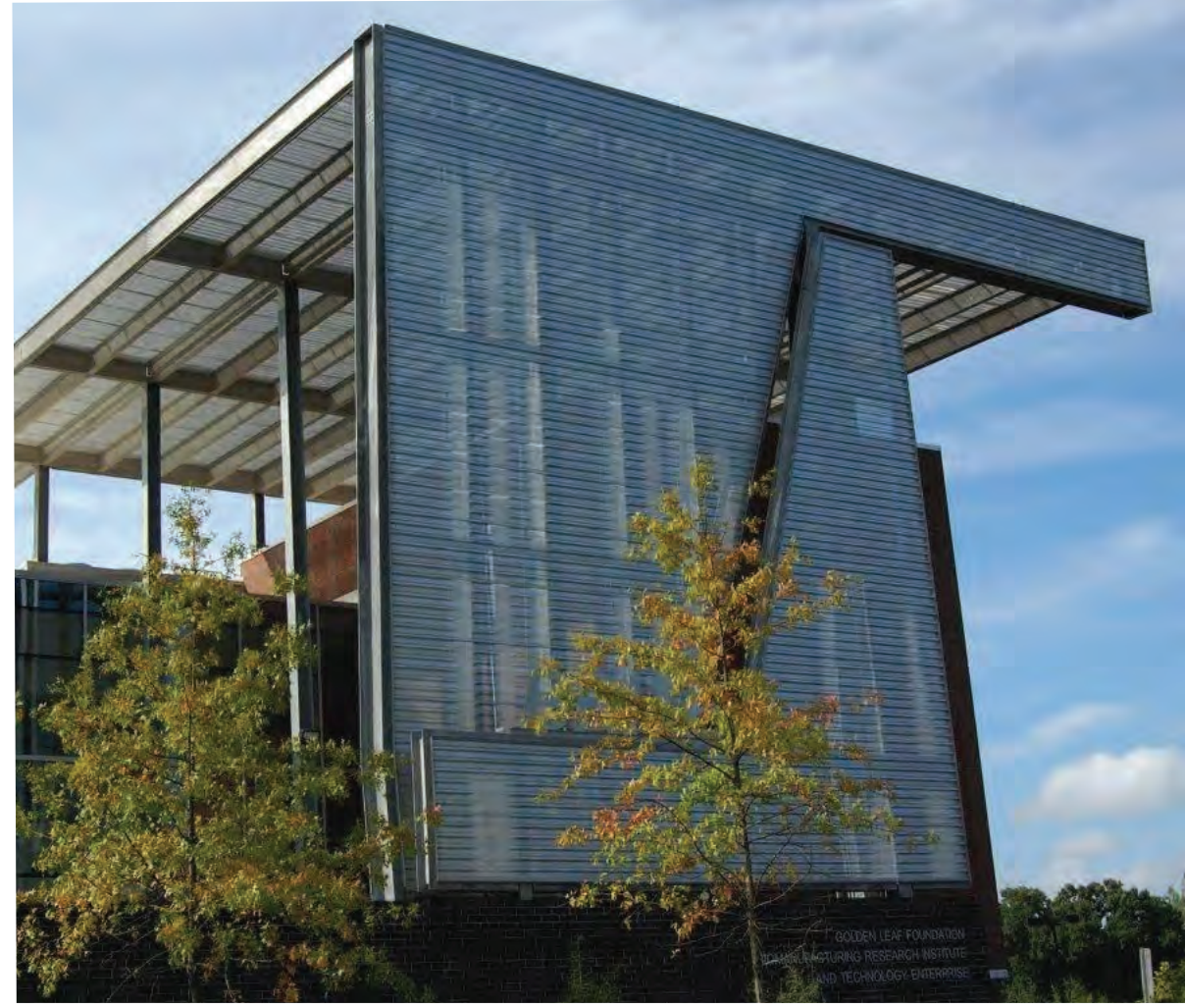
1. PERFORATED ZINC MECHANICAL SCREENS
