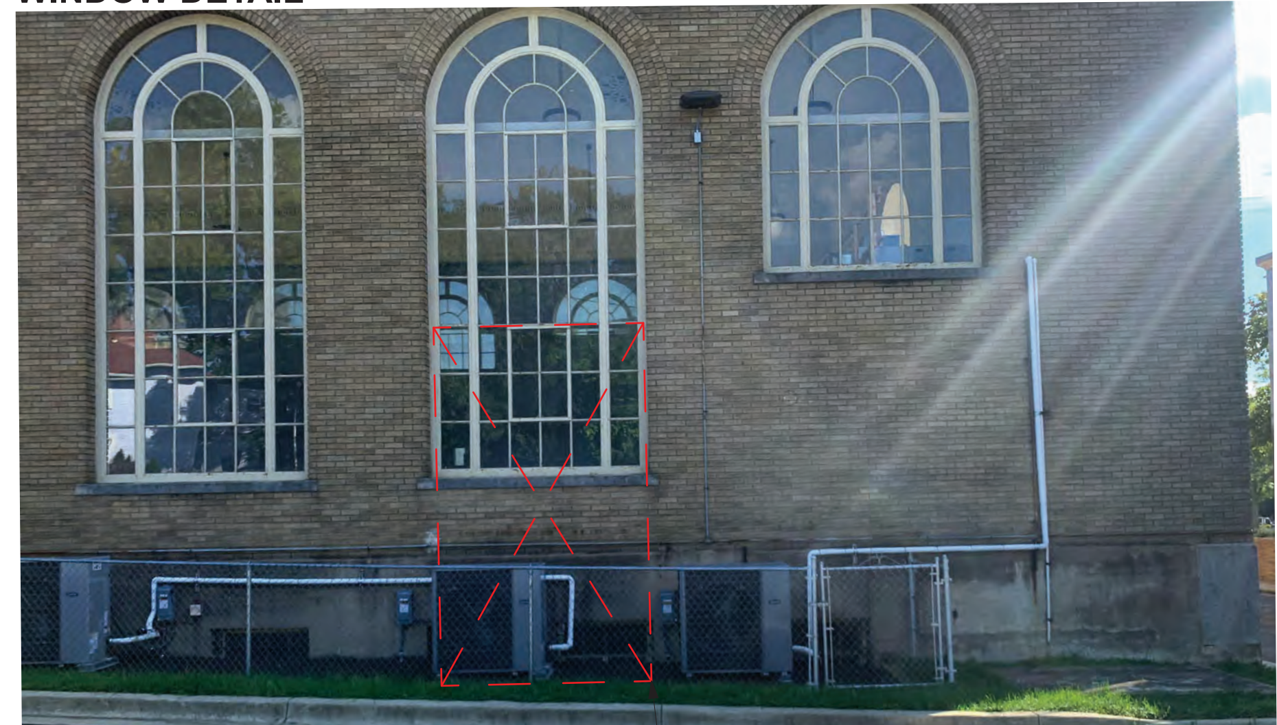
REPLACE WITH WINDOW FROM WILLOW AVENUE FACADE AND REMOVE SILL FOR ADDITION CONNECTOR
