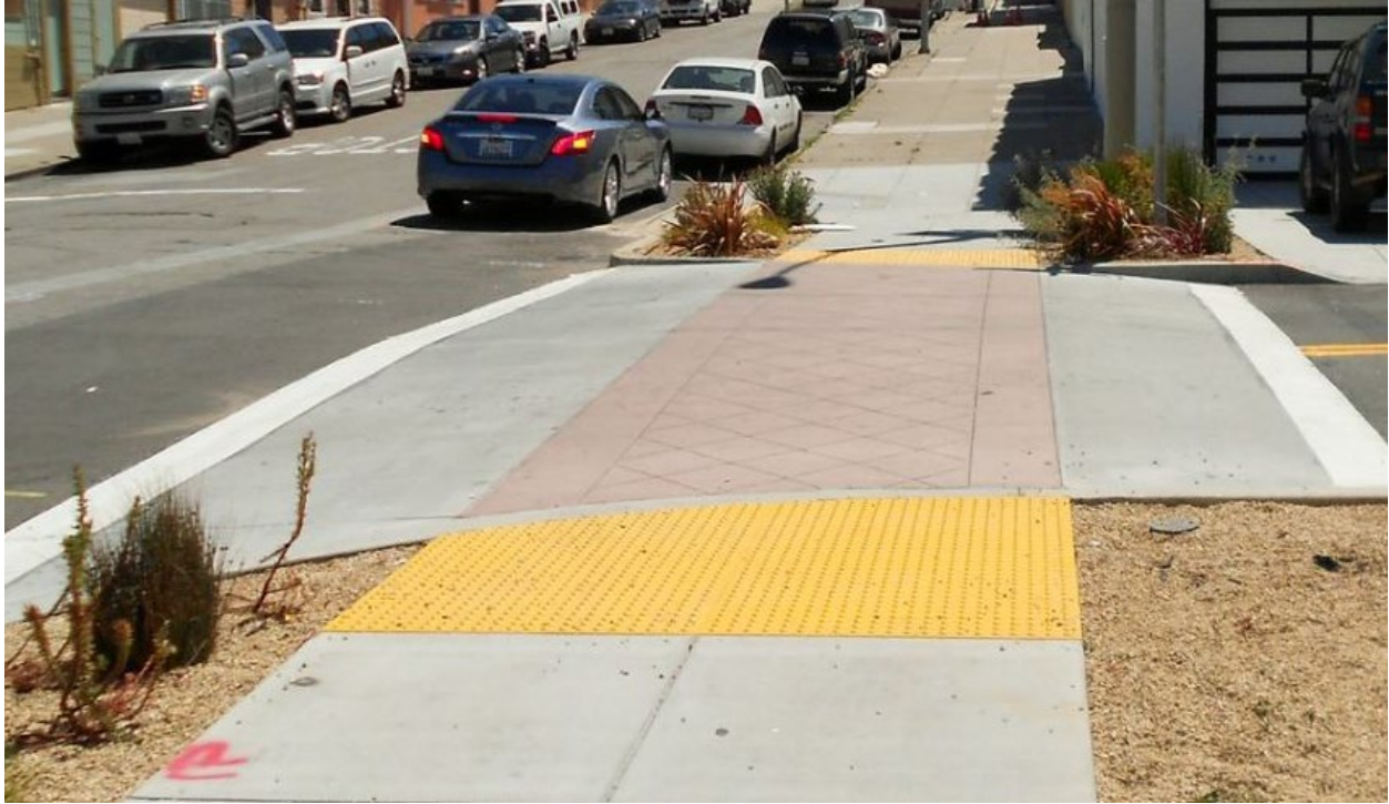
Figure 4: Driveway Crossing Flush with Sidewalk
