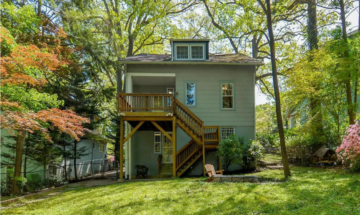
Figure 3: Existing rear elevation.
