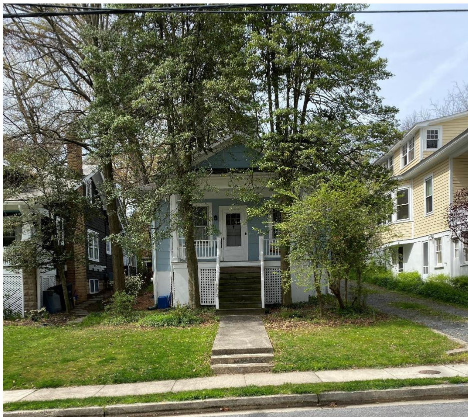
Figure 2: Front elevation of the subject property.
