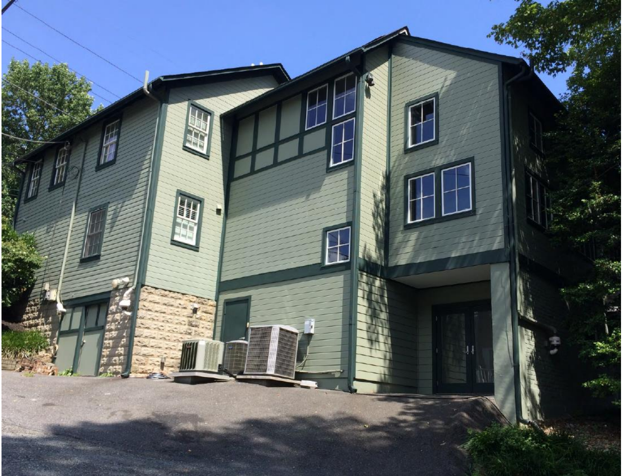
Fig. 4: Staff's July 2019 site visit photograph, showing three existing condensing units at the right side of the building.
