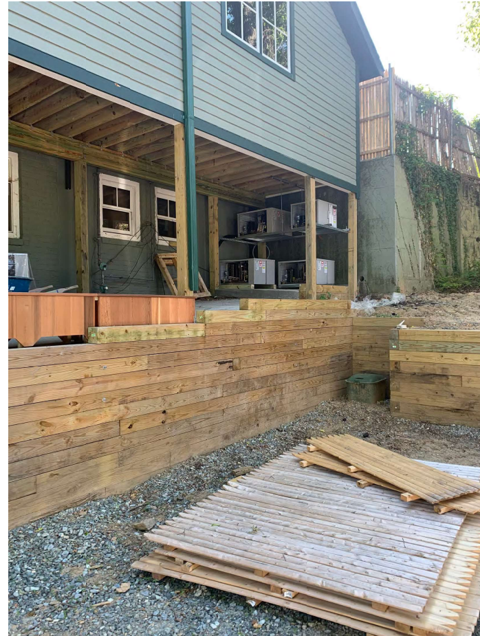
Existing conditions under addition
