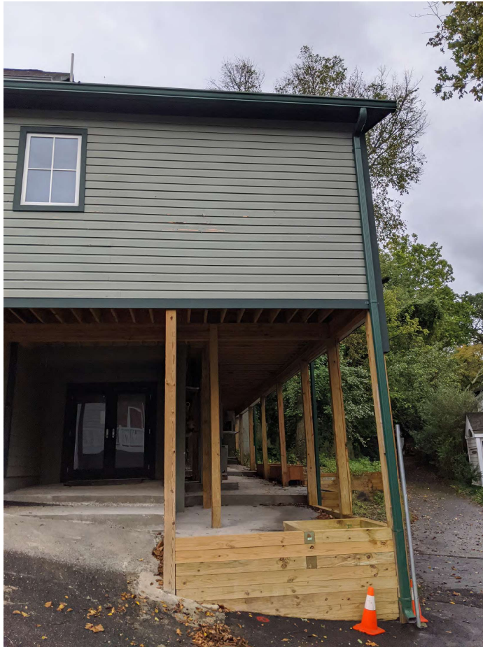
Existing conditions under addition
