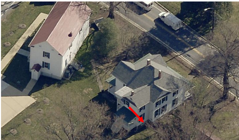
Figure 2: Aerial view of the rear of the Darby House (with Darby Store to the left). The red arrow points to the proposed location for the condenser units (heat pumps).
