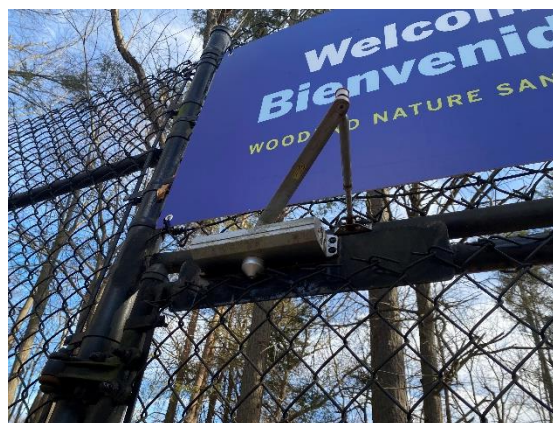
Existing Brierly Road Pedestrian Entrance
