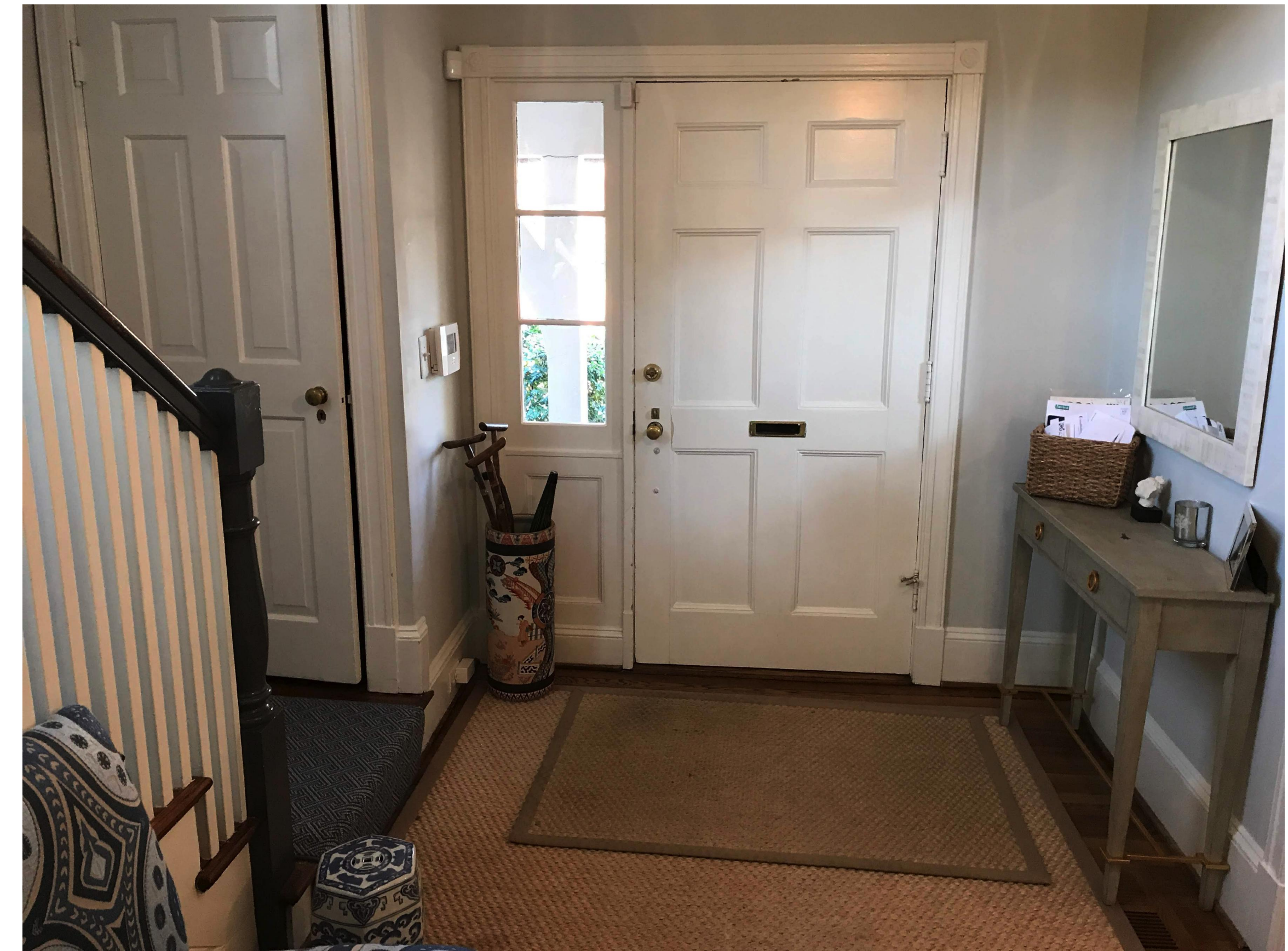
EXISTING FRONT DOOR
