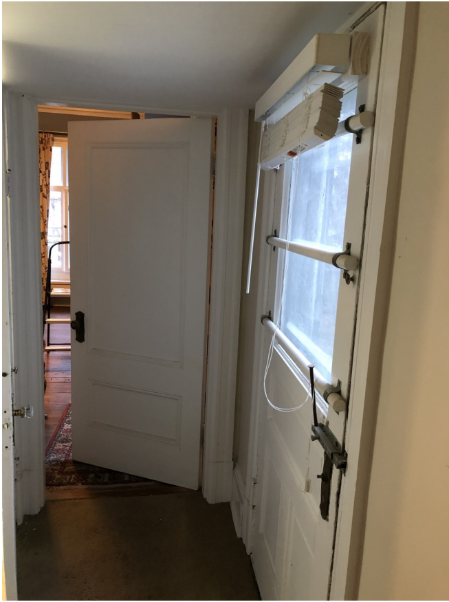
Existing Rear Hall Door
