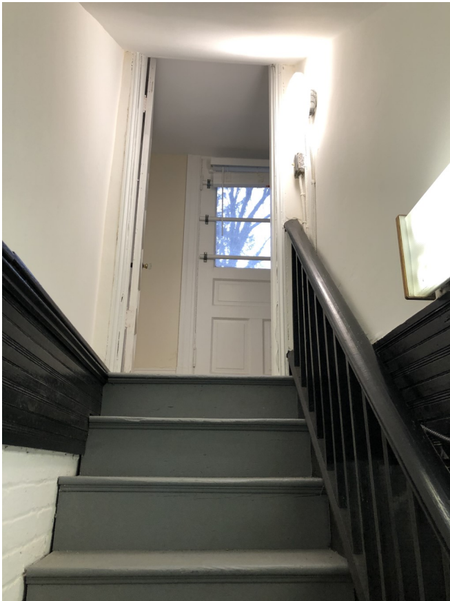
Existing Rear Hall Door as viewed from basement stairs.
