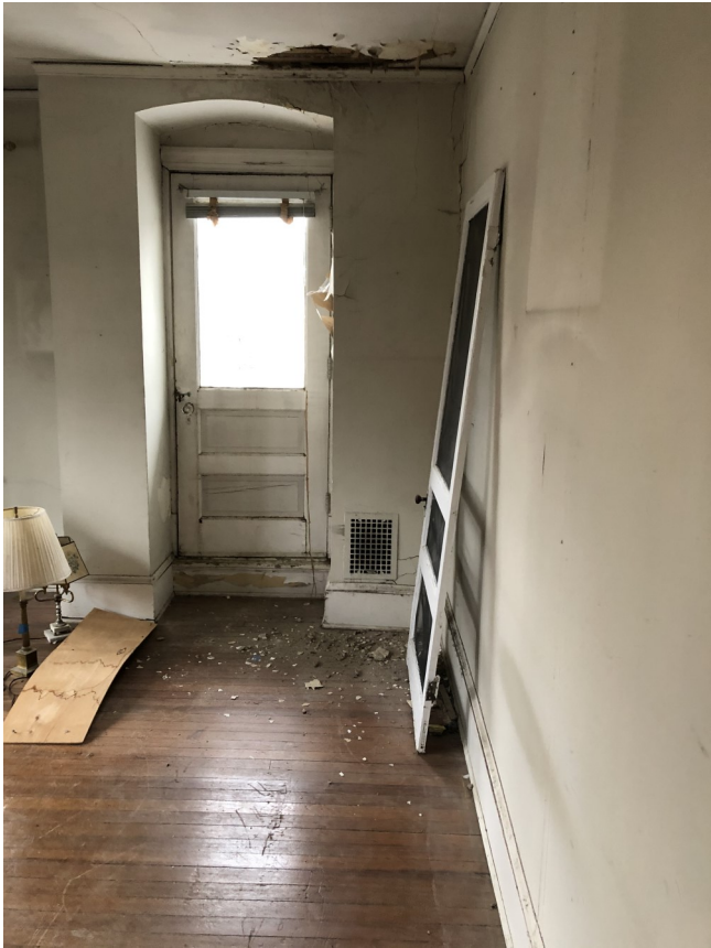
Existing Bedroom door to roof deck
