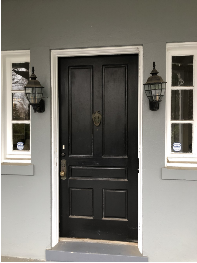
Existing Front door exterior
