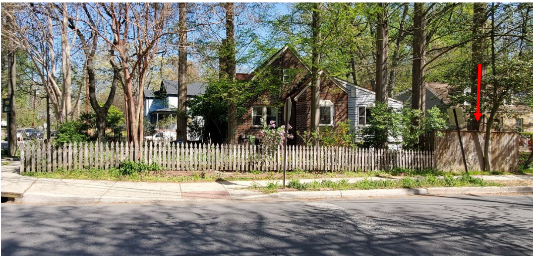
Figure 3: View of the south elevation from Elm Street showing the extant 3-tall picket fence (to be retained) and the remaining section of the 6'-tall privacy fence (red arrow) to be replaced with a picket fence, 2023. Source: Montgomery Planning.
