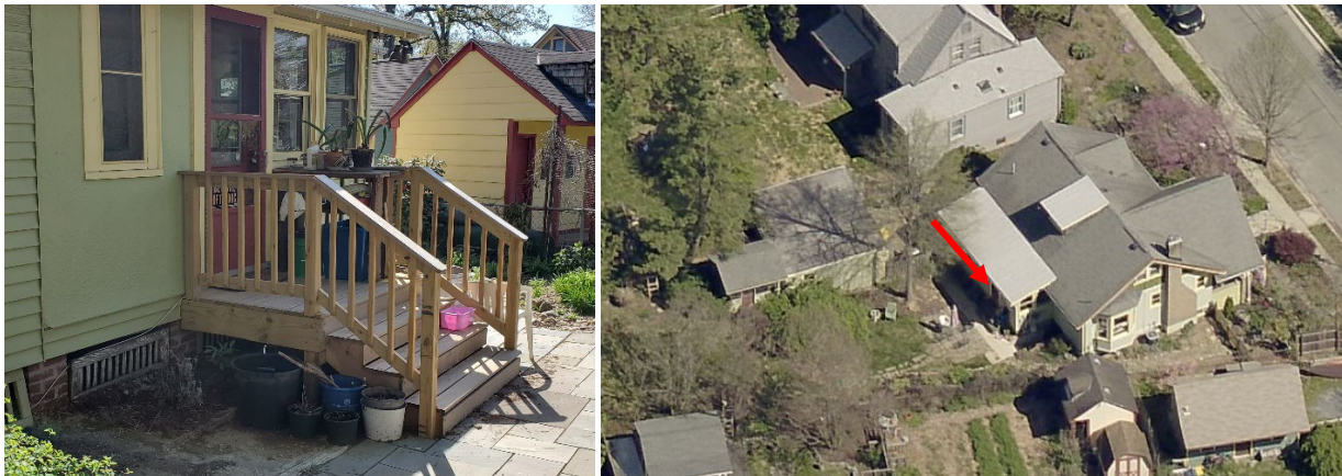
Figure 3: View of the new wood stair, railing, and landing, 2023 (left), and aerial view of the house, 2021 (right). The red arrow points to the location of the installed stair.
