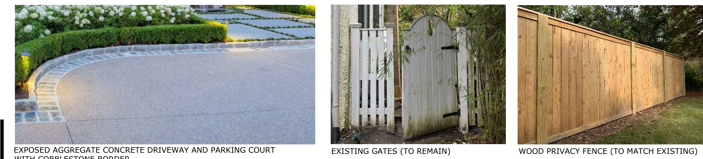
EXPOSED AGGREGATE CONCRETE DRIVEWAY AND PARKING COURT WITH COBBLESTONE BORDER | EXISTING GATES (TO REMAIN) | WOOD PRIVACY FENCE (TO MATCH EXISTING)
