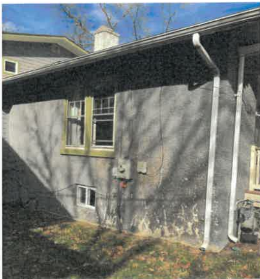
Seavey Utility Side Before Installation
