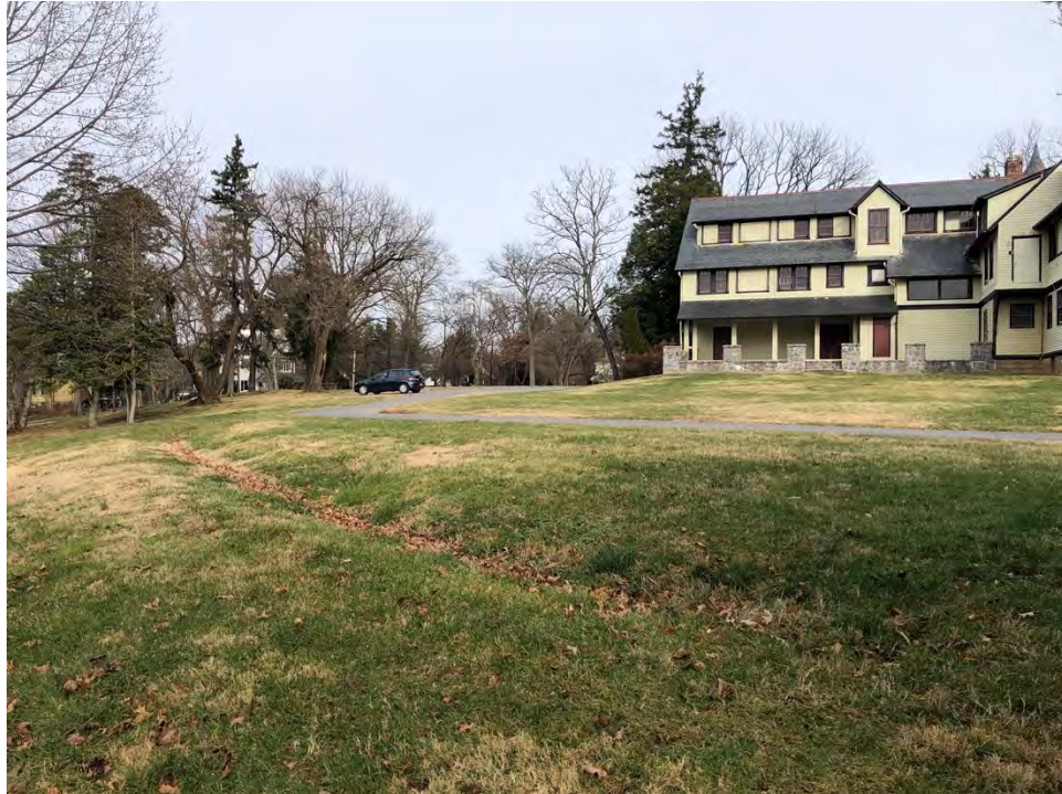
Figure 2.10: View of Modern Drainage Feature Southwest of the Brainard Warner House, Facing North .
