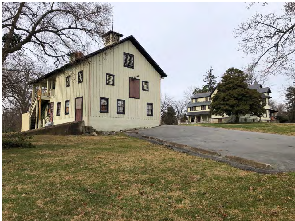
Figure 2.7: View of Carriage House at South Side of Warner Circle Park, Facing Northwest.
