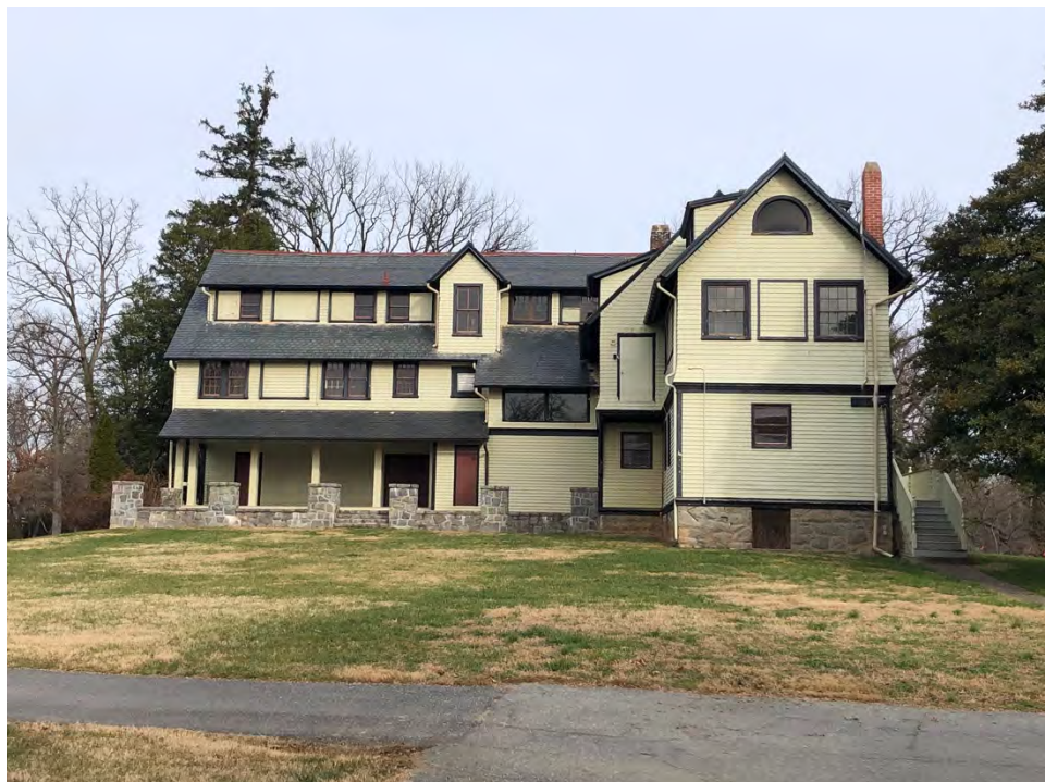
Figure 2.9: View of South Façade of Brainard Warner House and Former Location of 1956 Nursing Home Addition, Facing North.
