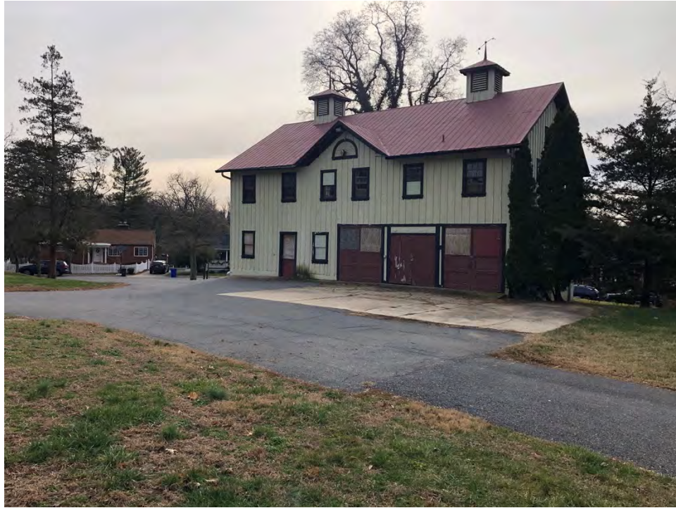
Figure 2.8: View of Carriage House at Warner Circle Park, Facing South-Southeast.
