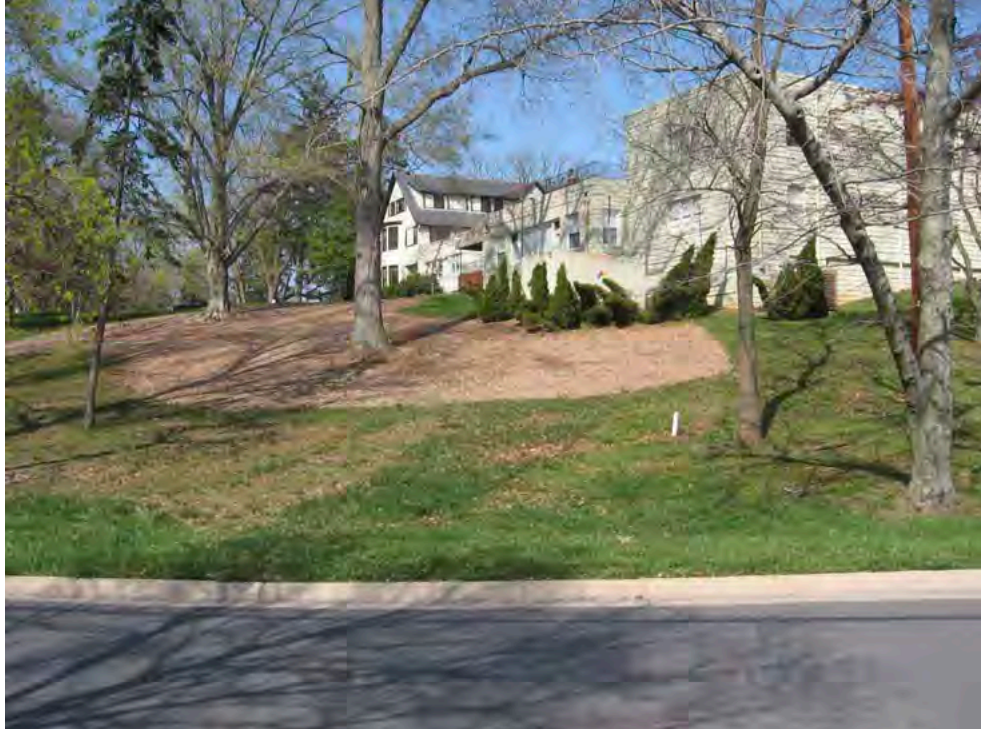
Figure 3.1: View of Former Addition on Southern Side of Warner Mansion Photographed by ca. 2010, Facing Northeast (from Fischler and French 2010:Figure 2.3).
