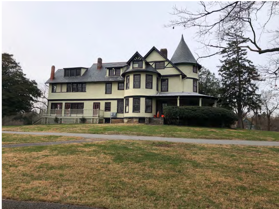
Figure 2.5: View of East Façade of the Brainard Warner House, Facing West.
