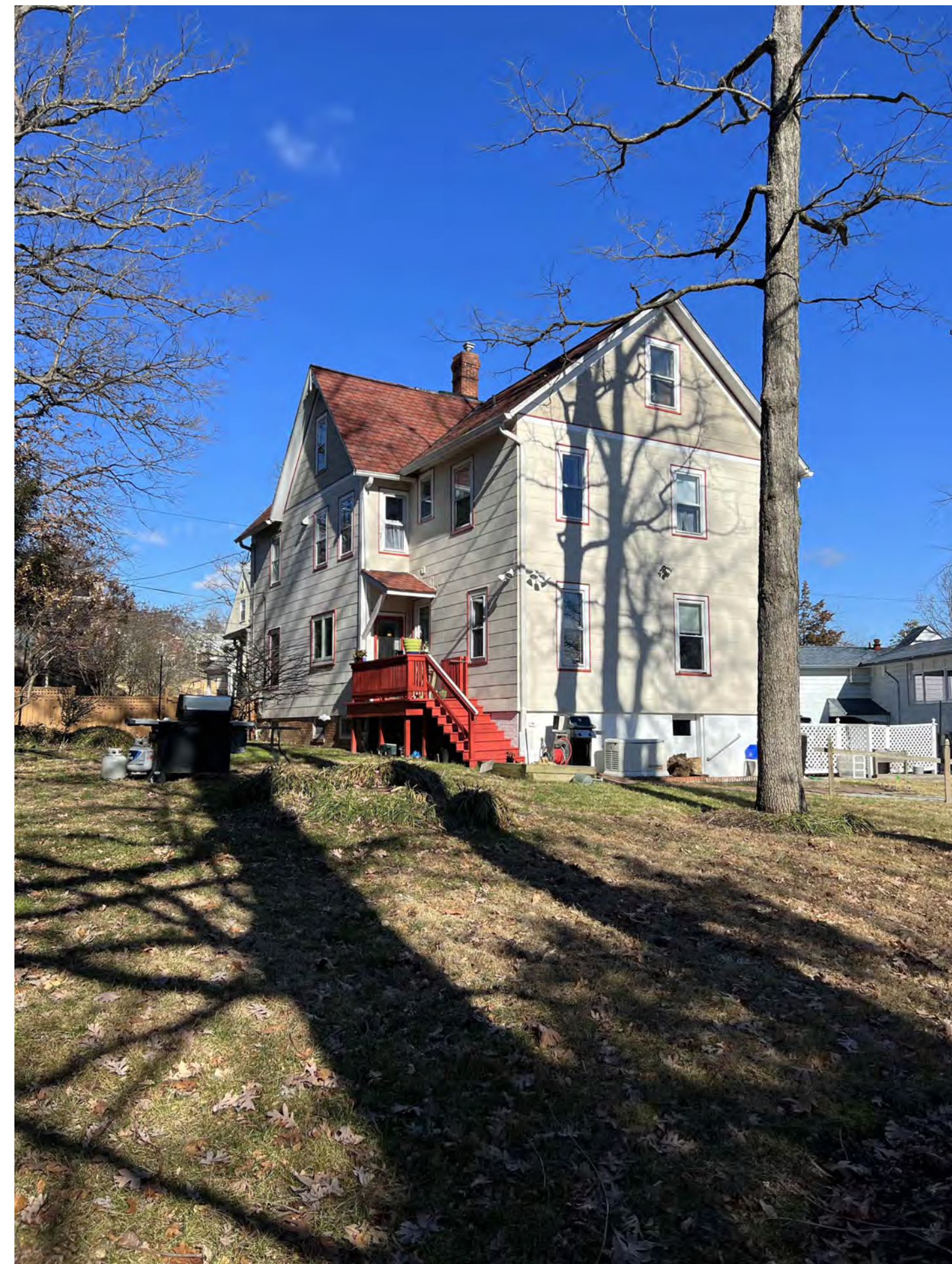
Existing conditions looking at South(Back) and West(Side) Facades
