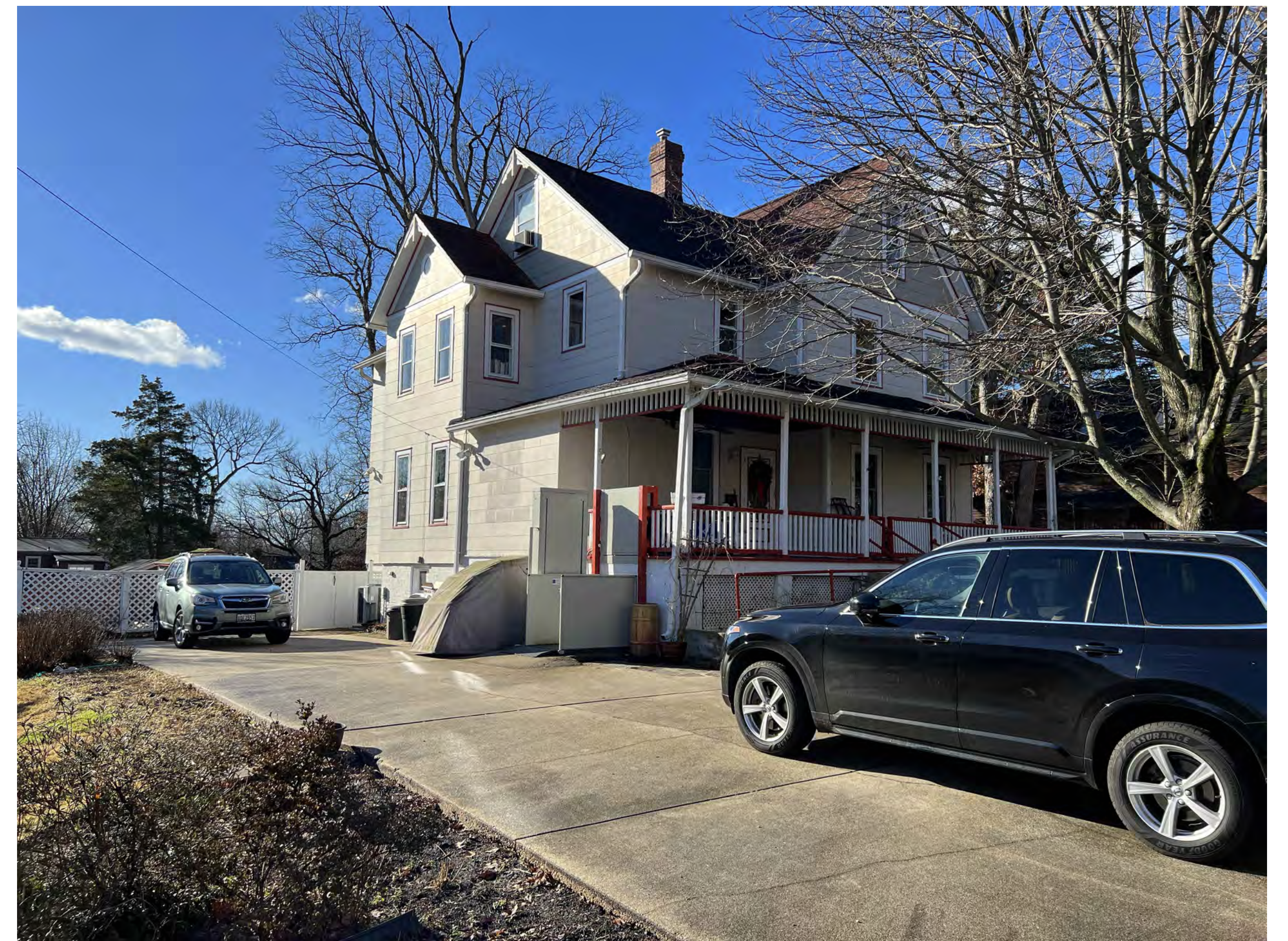
Existing conditions looking at North(Front) and East(Side) Facades
