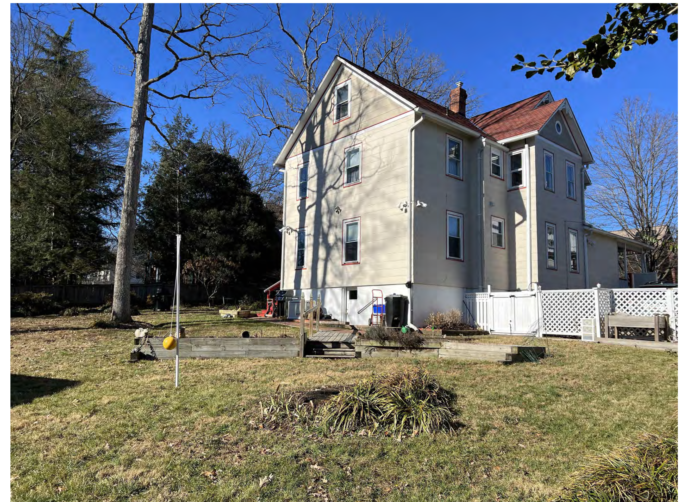
Existing conditions looking at South(Back) and East(Side) Facades
