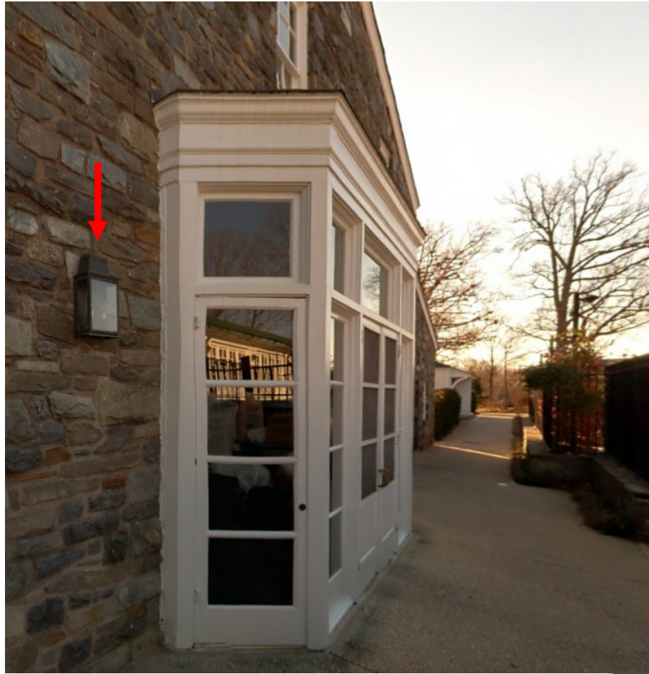
Existing fixtures to be replaced
