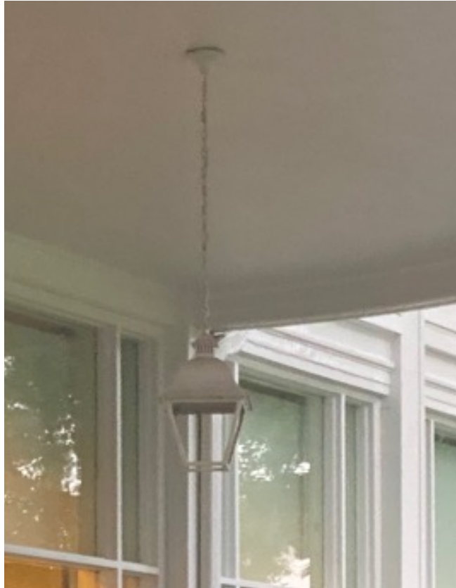
Existing fixture to be replaced
