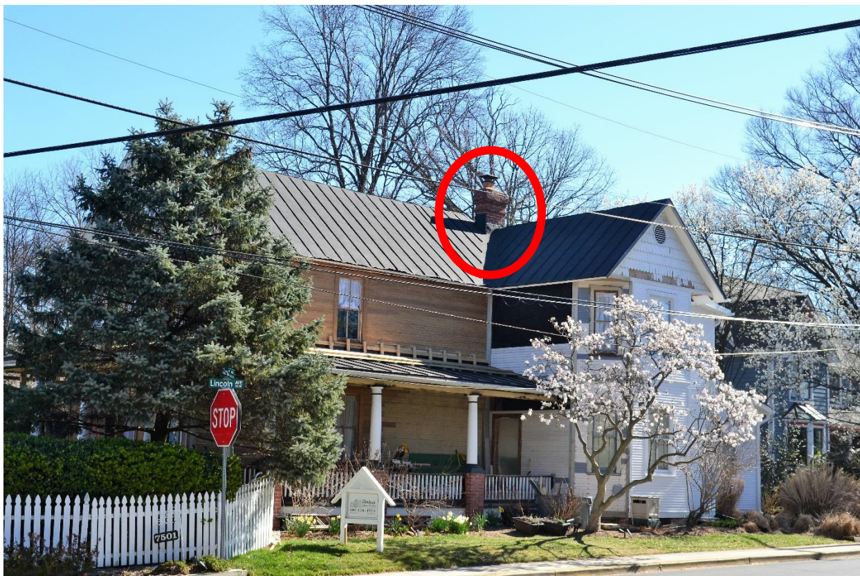
Figure 3: The subject property from the northwest (chimney to be removed circled).
