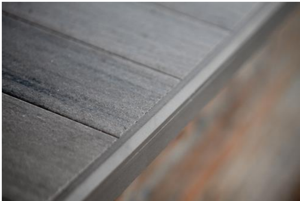
Figure 2: Detail of the chamfer nosing installed.
