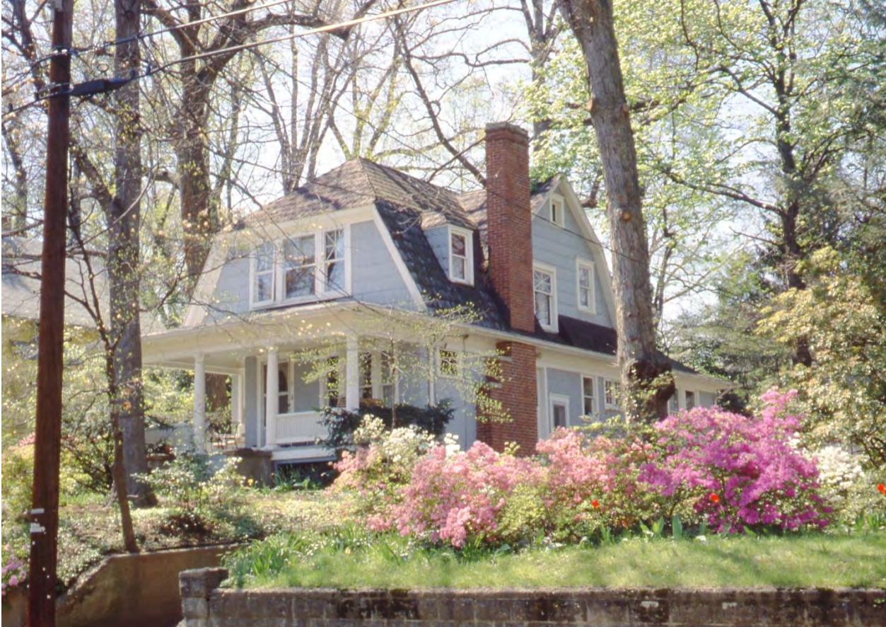
Figure 2: Undated photo of the subject property before the 2008 roof replacement.
