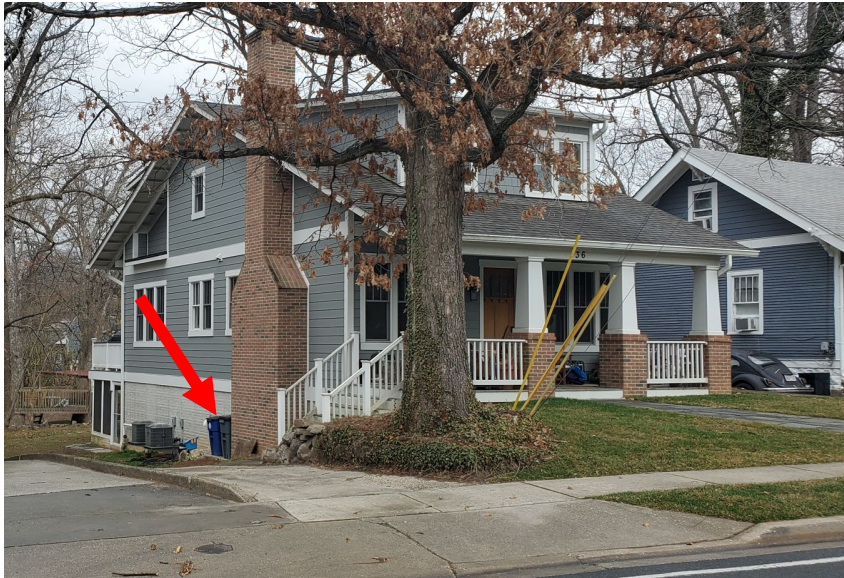
Figure 4: View of the chimney on the north elevation, 2023. The red arrow points to the current location of the trashcan pad.
