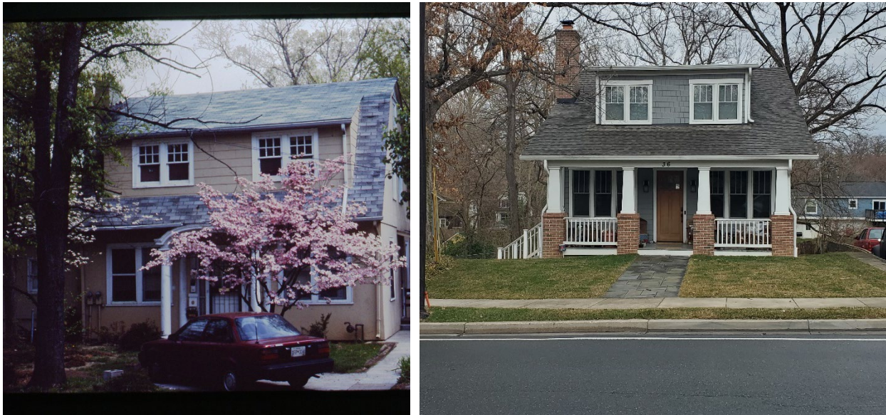
Figure 2: View of the former contributing house demolished in 2012, undated (left), and view of the façade of the non-contributing house from Philadelphia Avenue, 2023 (right).
