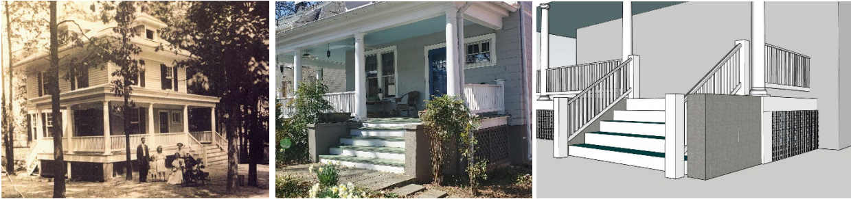
Figure 2: View of the facade of the house, 1909 (left) and 2023 (center), and model of the proposed stair balustrade (right). Note the original demolished stair railing extended from the center of the column to a newel post. Source: Property Owner and Montgomery Planning.
