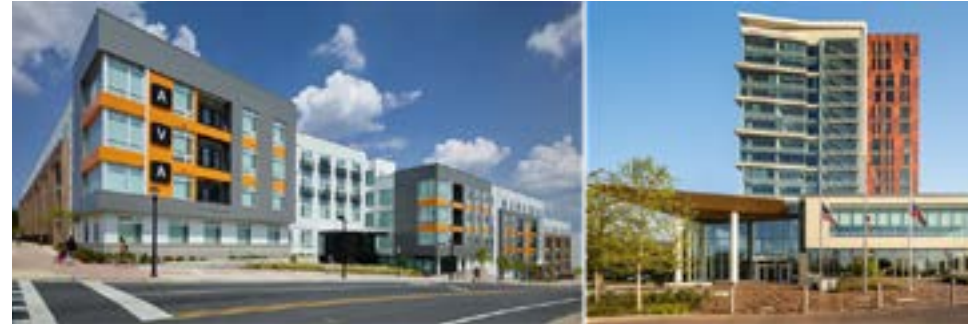
Clockwise from top left: Solaire Wheaton, Arrive Wheaton, The George, M-NCPPC HQ, AVA Wheaton
