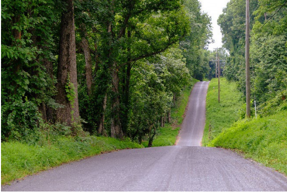
Rollercoaster alignment and steep embankments along the edge of the road
