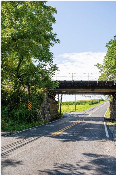
Looking south at the railroad bridge crossing Beallsville Road
