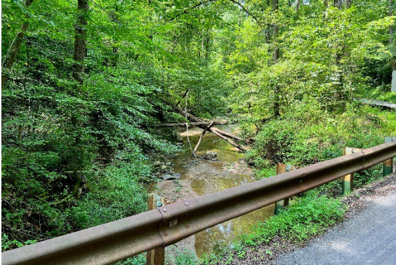
Looking into Seneca Creek at the southernmost narrow bridge crossing
