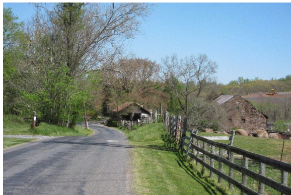
Looking north on Martinsburg Road towards the Stone Bank Barn
