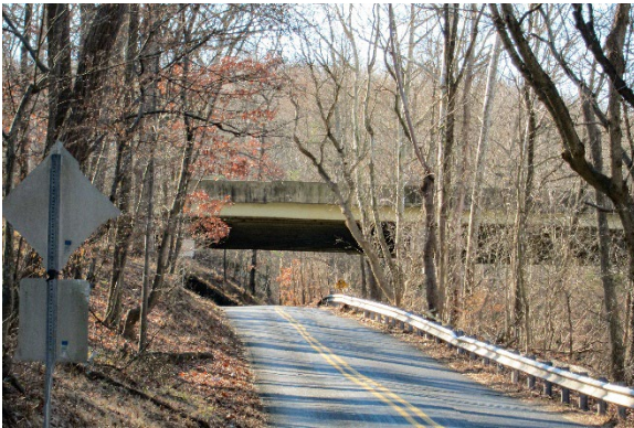
Game Preserve Road running underneath I-270
