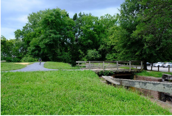
C&O Canal Towpath adjacent to Lock #23
