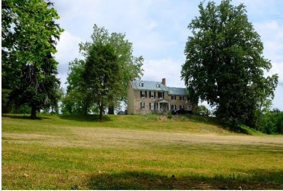
Elton is located midway along Elton Farm Road on the north side of the road
