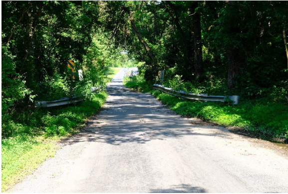
View looking east towards West Willard Road of the two one-lane bridges crossing the Horsepen Branch and its tributary
