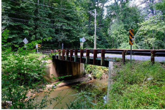
One-lane bridge over the Watts Branch
