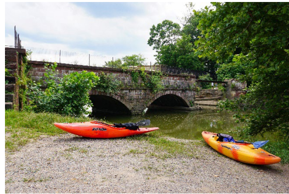
Seneca Creek Aqueduct
