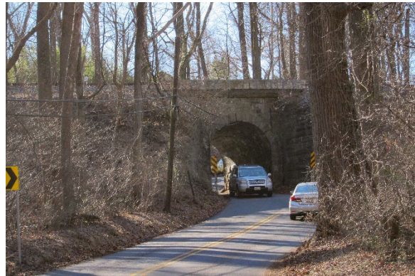
One-lane railroad underpass on Game Preserve Road
