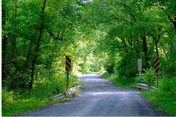
The southernmost one-lane bridge on Sycamore Landing Road
