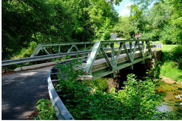
Truss bridge over Dry Seneca Creek
