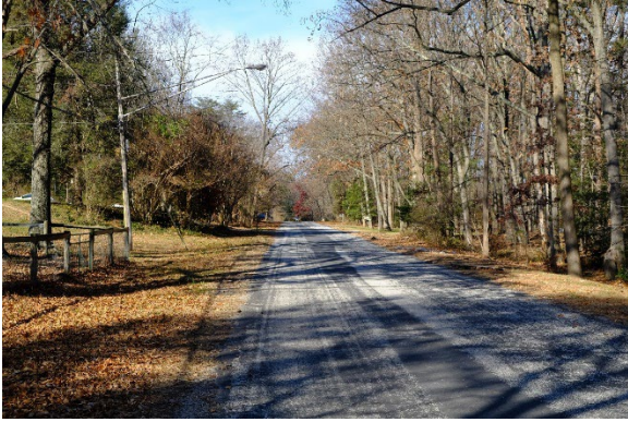
Looking northwest on Aitcheson Lane
