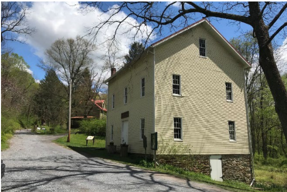
Looking east on Hyattstown Mill Road towards the Hyattstown Mill Complex on the right with the park gate in the distance
