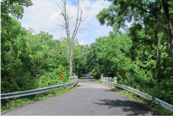
Looking east on Schaeffer Road towards the one-lane pipe bridge over Little Seneca Creek
