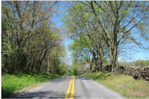
Looking north towards the intersection with Martinsburg Road (Seneca Sandstone wall on the east side)
