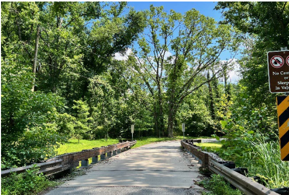
One-lane bridge crossing over Muddy Branch
