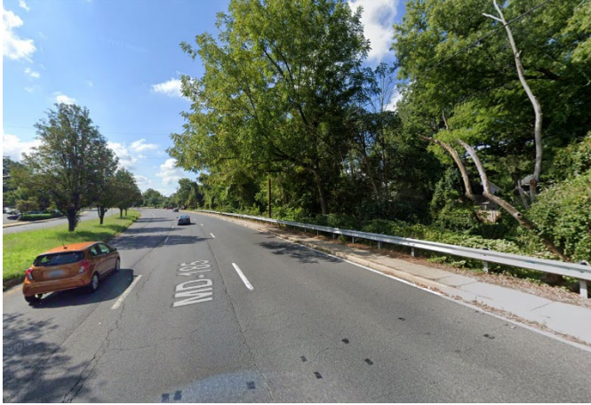
Guardrail behind sidewalk along Connecticut Avenue in Aspen Hill. Photo Credit: Google Maps
