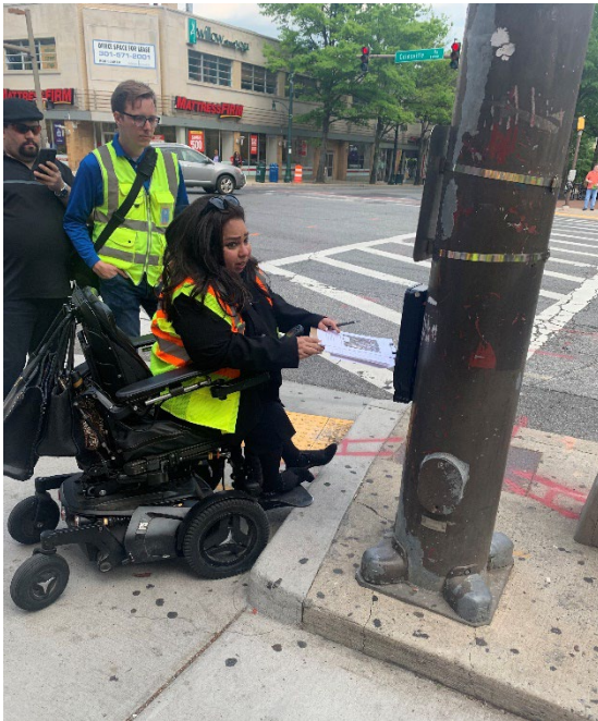
This pedestrian is unable to reach an APS in Downtown Silver Spring because the push button is located on a raised surface that her mobility device cannot navigate.
